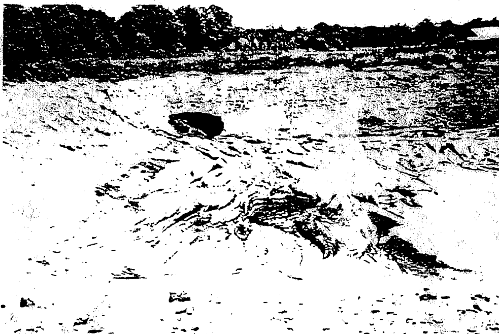
FIGURE 8. Sinkhole collapse under a hog waste lagoon in Logan County on April 29, 1991. The plastic liner under the lagoon extended across the bottom and 4 feet up the sides. The collapse occurred above the liner when the lagoon was 12.8 feet deep.
