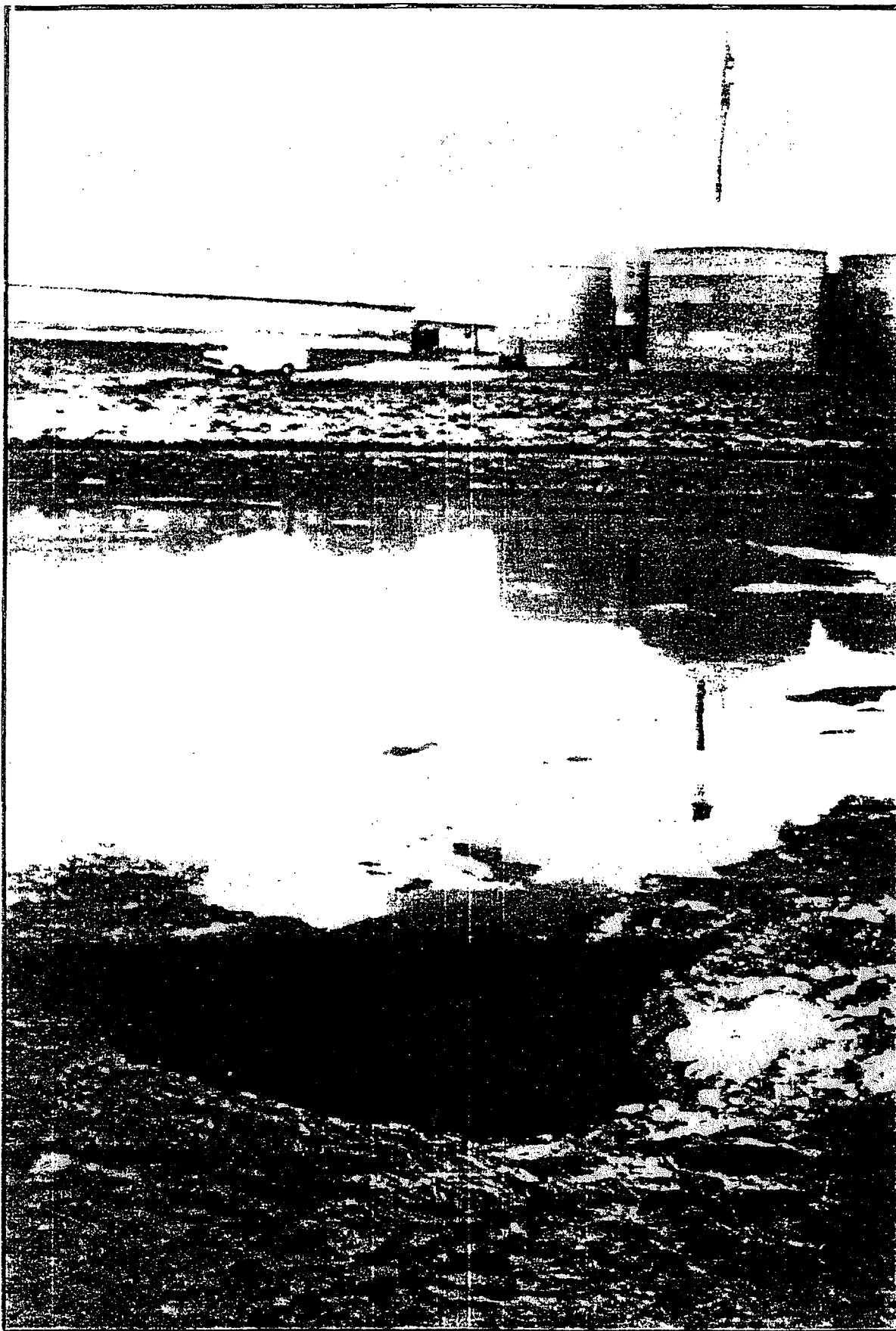
FIGURE 3. Sinkhole collapse under hog waste lagoon in March 1984 on Barren County, Kentucky. Approximately 2.4 million gallons of hog waste sank into the karst aquifer in less than 5 hours. Impoundment of water and concentration of surface runoff are the leading causes of sinkhole collapses in the karst areas of Kentucky. Photograph by Kentucky Division of Water.
