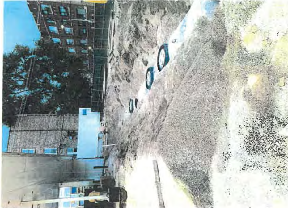
PROJECT: East West Properties, LLC-Ashland Ave PHOTOGRAPH #22 DATE: 9/26/23 VIEW: South DESCRIPTION: Backfilling Tank Excavation with Gravel
