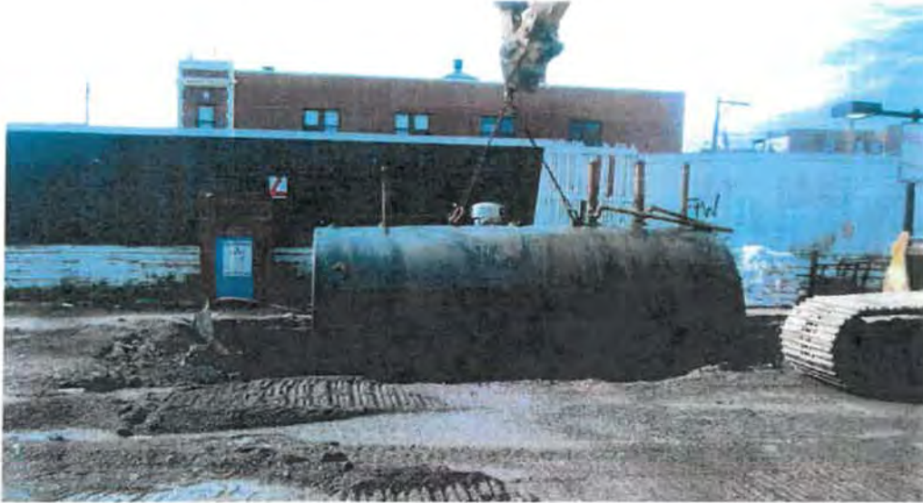
PROJECT: East West Properties, LLC-Ashland Ave PHOTOGRAPH #3 DATE: 9/6/23 VIEW: South DESCRIPTION: Removing Kerosene Tank.
