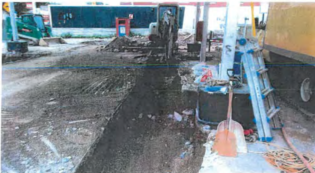
PROJECT: East West Properties, LLC-Ashland Ave PHOTOGRAPH #8 DATE: 9/7/23 VIEW: South DESCRIPTION: Piping Removal.
