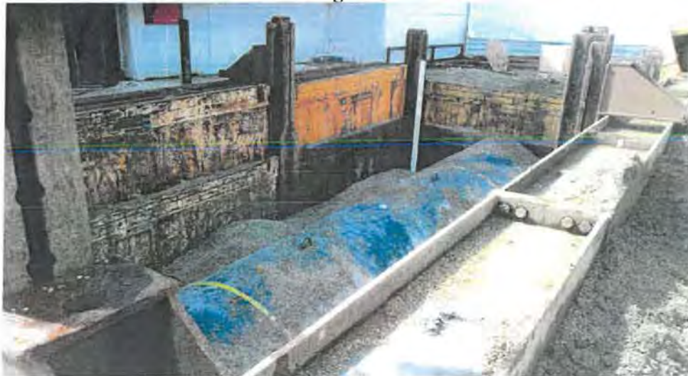
PROJECT: East West Properties, LLC-Ashland Ave PHOTOGRAPH #22 DATE: 9/26/23 VIEW: South DESCRIPTION: Backfilling Tank Excavation with Gravel
