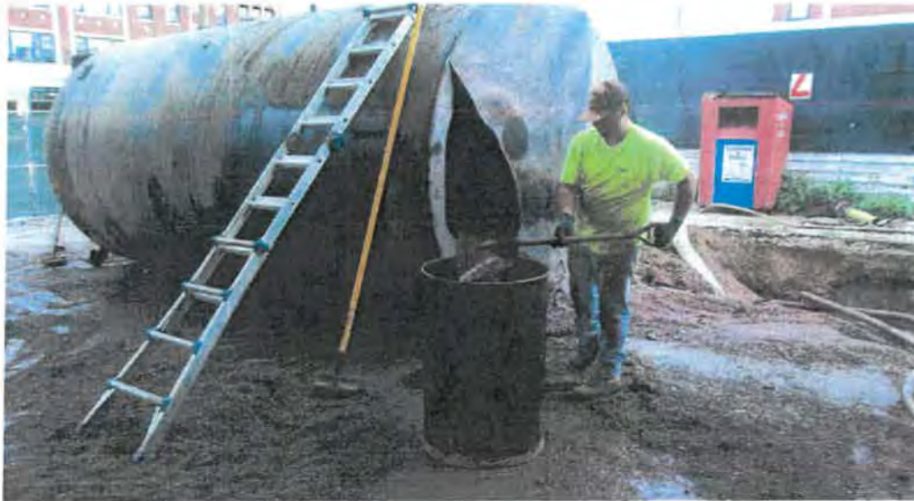
PROJECT: East West Properties, LLC-Ashland Ave PHOTOGRAPH #5 DATE: 9/6/23 VIEW: Southeast DESCRIPTION: Cleaning Out Kerosene Tank.
