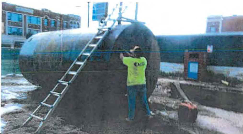
PROJECT: East West Properties, LLC-Ashland Ave PHOTOGRAPH #4 DATE: 9/6/23 VIEW: Southeast DESCRIPTION: Cutting Open Kerosene Tank.
