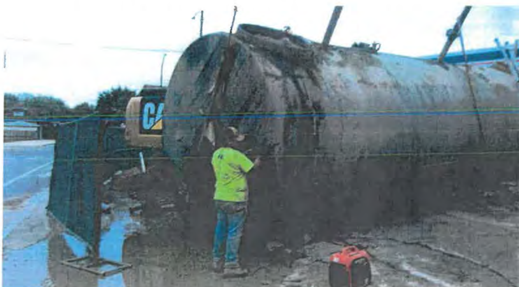
PROJECT: East West Properties, LLC-Ashland Ave PHOTOGRAPH #14 DATE: 9/7/23 VIEW: East DESCRIPTION: Cutting Open Gasoline Tank.
