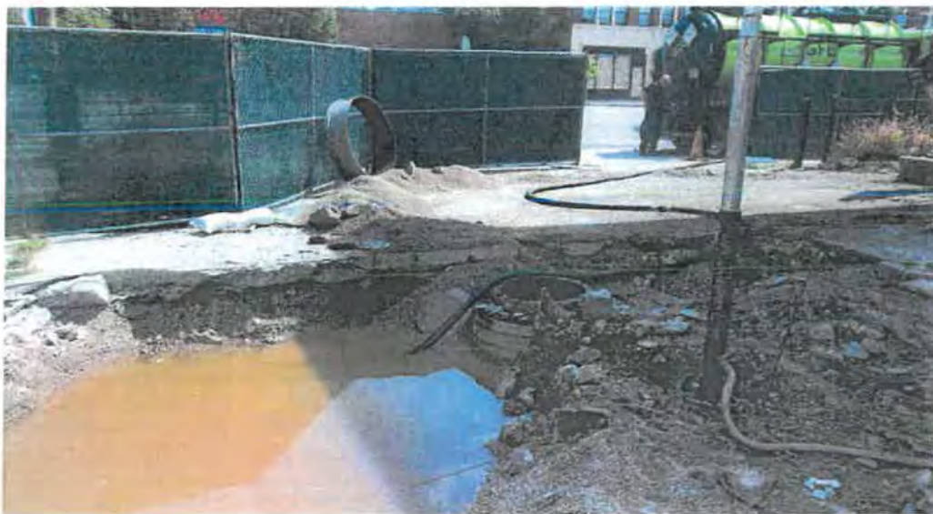
PROJECT: East West Properties, LLC-Ashland Ave PHOTOGRAPH #6 DATE: 9/6/23 VIEW: East DESCRIPTION: Pumping Water out of excavation around Gasoline Tank.
