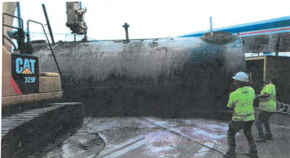
PROJECT: East West Properties, LLC-Ashland Ave PHOTOGRAPH #13 DATE: 9/7/23 VIEW: East DESCRIPTION: Removing Gasoline Tank.
