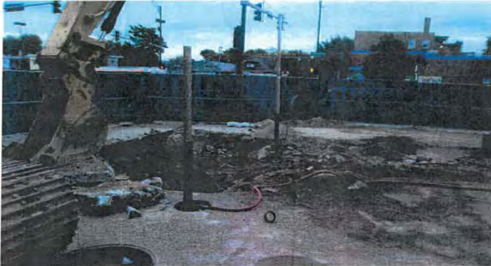
PROJECT: East West Properties, LLC-Ashland Ave PHOTOGRAPH #7 DATE: 9/7/23 VIEW: East DESCRIPTION: Blowing Down Gasoline Tank.
