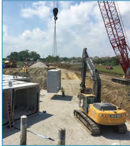
Construction on the bridge replacement on Steger Road over Jackson Creek.
