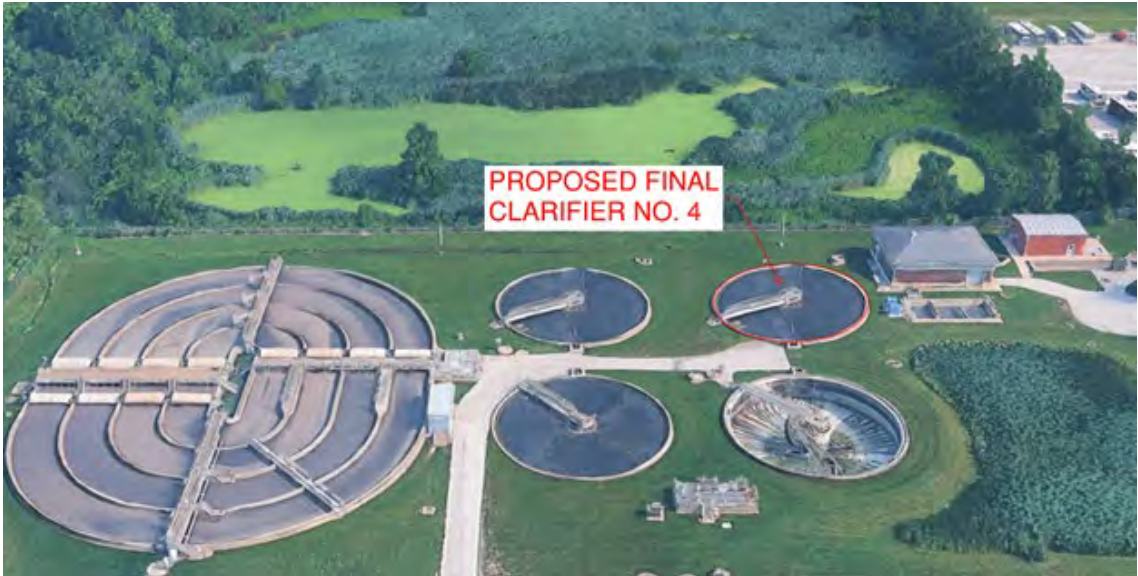
Figure 2 - Phase 1: Final Clarifier No. 4
