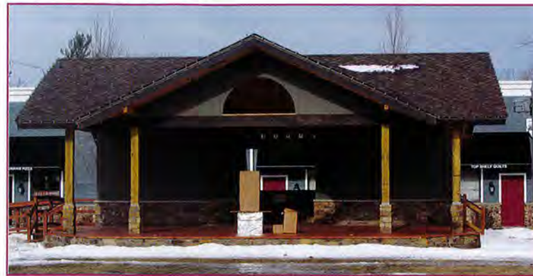
Finishing work on Breidert Green stage continues on schedule.
