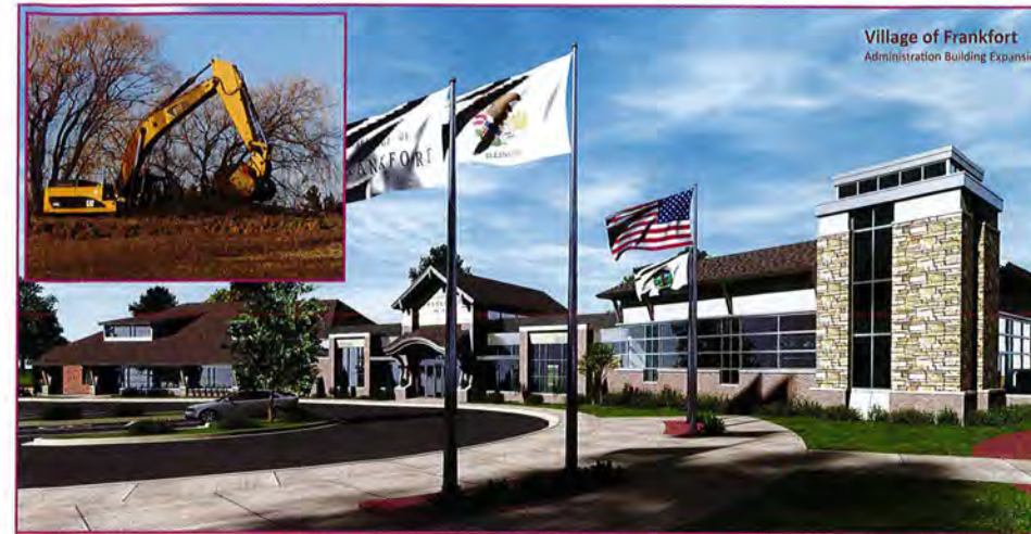
The excavator (inset) has begun site excavation for the new Village board room.
