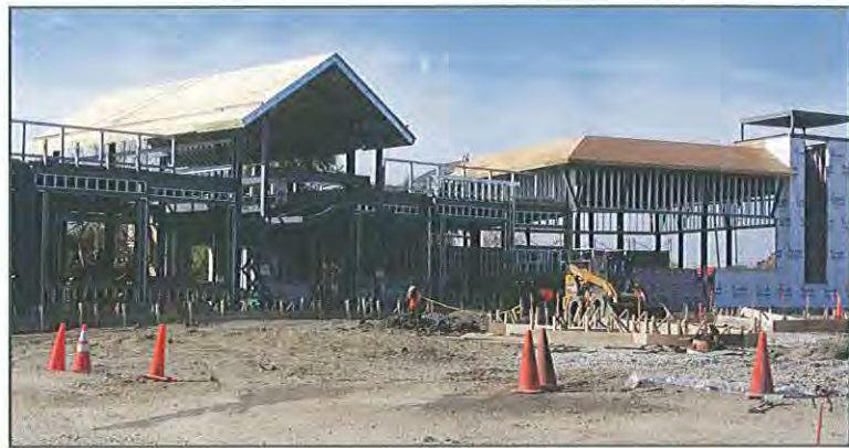
The village hall expansion project continues to progress well.
