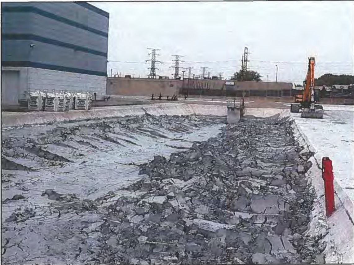
Photograph 3.6 – Dewatered lime sludge solids ready to be excavated for landfill disposal
