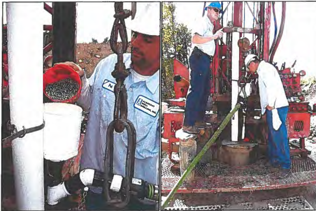
Photographs 7.7 and 7.8- Hopper attached to tremie pipe; well casing on left
