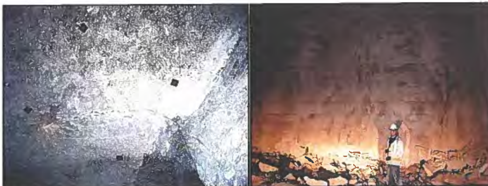
Photographs 11.5 and 11.6 – (left): Ceiling showing J1 and J2 joint sets and roof bolts
