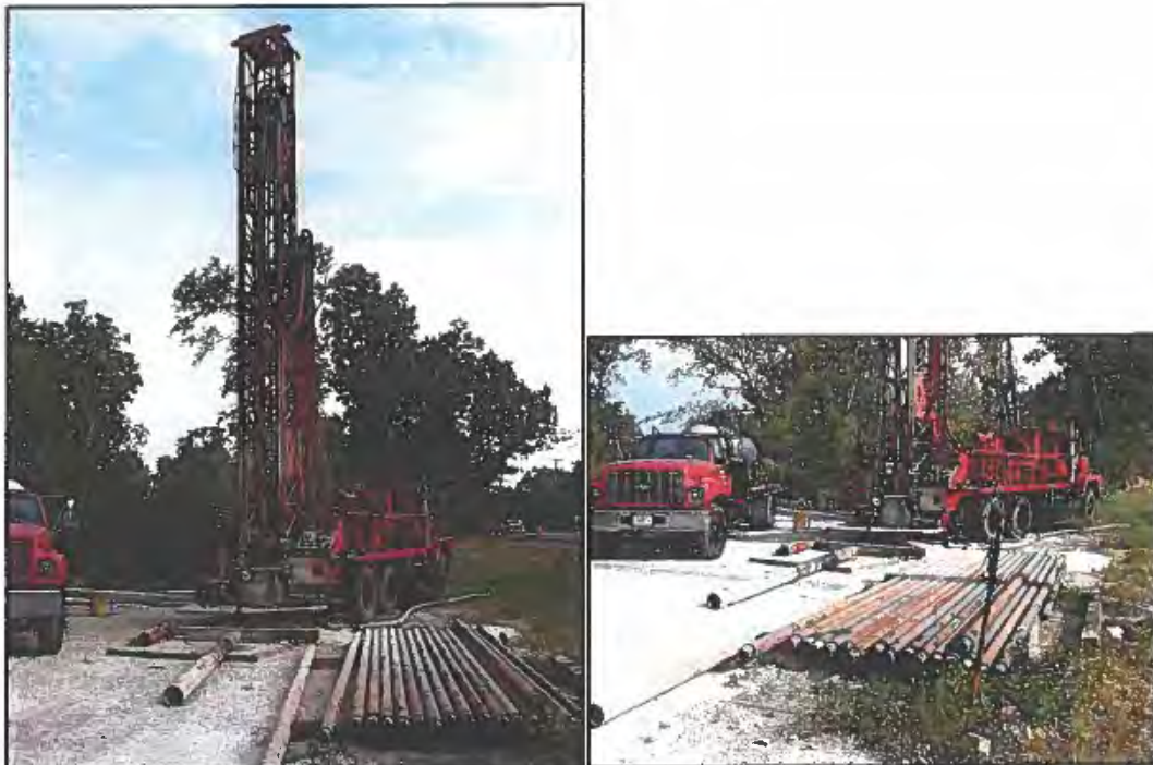
Photographs 7.1 and 7.2- Drill rig used for MW construction and tanker truck
