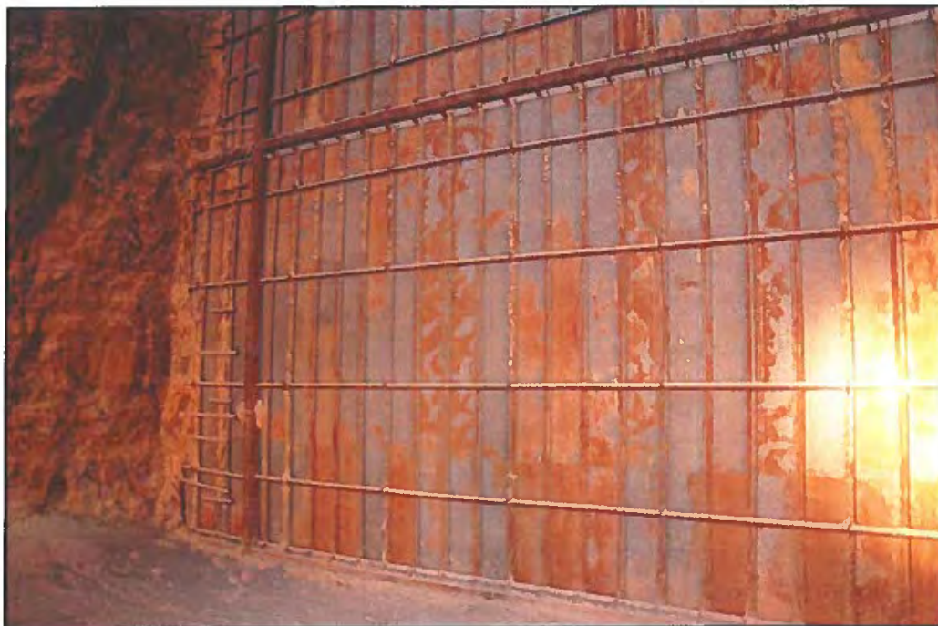
Photograph 11.22 - Completed stopping
