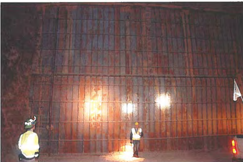
Photographs 11.23 - Completed stopping
