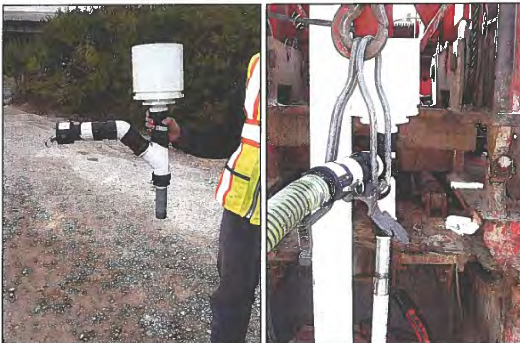
Photographs 7.3 and 7.4- Hopper used for placement of annular materials
