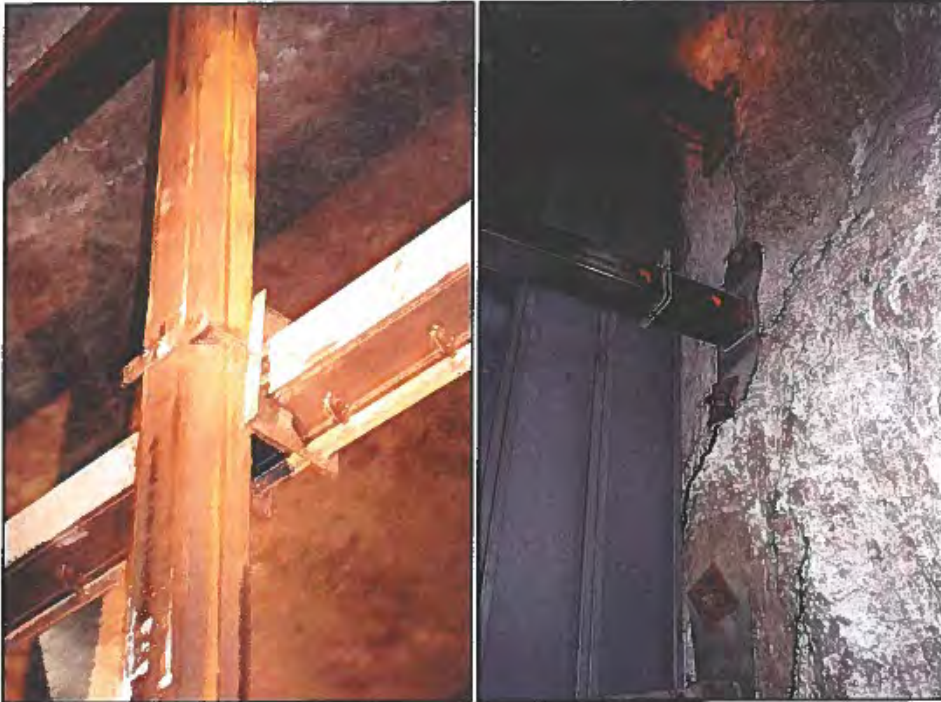
Photographs 11.18 and 11.19 - Bracing ties and rib bolts
