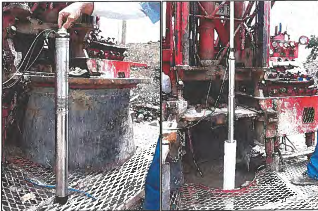
Photographs 7.11 and 7.12- Grundfos submersible pump
