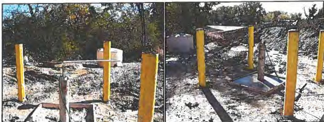
Photographs 7.13 and 7.14- Wellhead with pump discharge line
