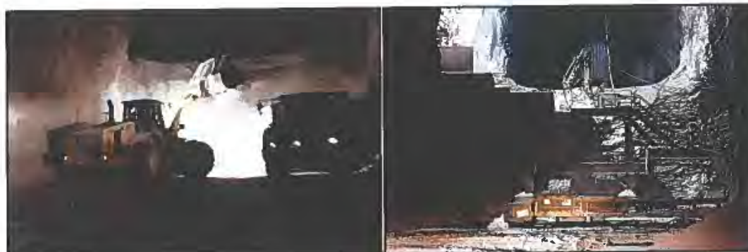
Photographs 11.7 and 11.8 - Loading shot rock into dump truck and rock crusher
