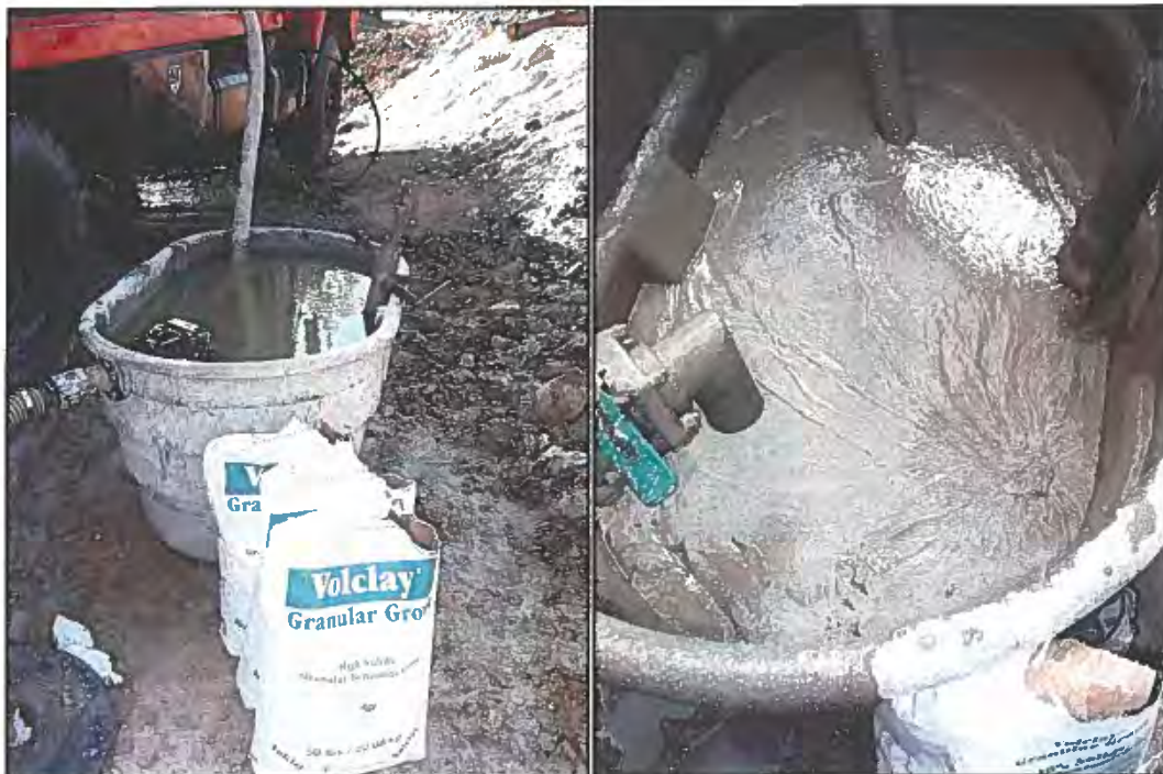
Photographs 7.9 and 7.10- Bentonite grout and mixing tank
