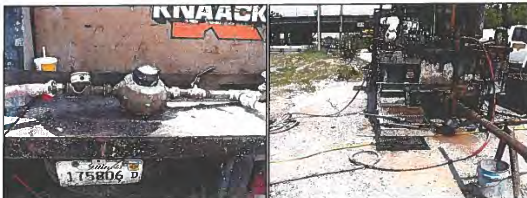
Photographs 5.11 and 5.12 - Pressure gauge and packer assembly attachment to well
