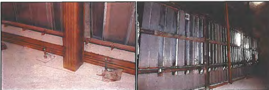
Photographs 11.16 and 11.17 - Bracing showing floor bolts and connection to panels
