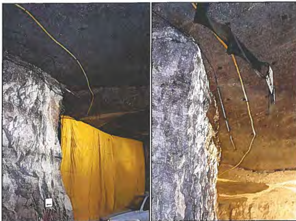
Photographs 11.3 and 11.4 – Pillar and ceiling with yellow air flow diversion blanket
