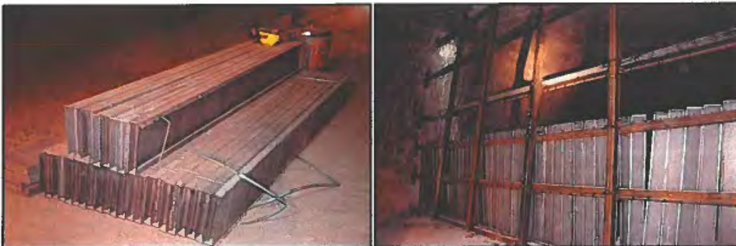
Photographs 11.14 and 11.15 - Stoppings steel panels and heavy duty braces
