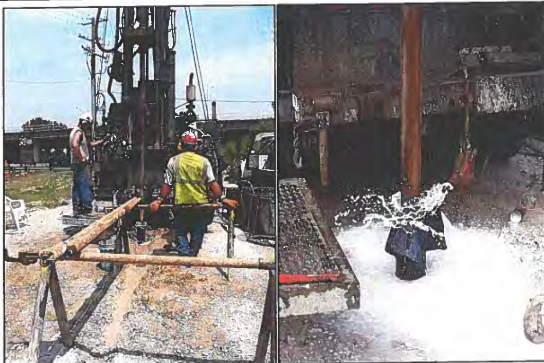
Photographs 5.2 and 5.3 - Wireline coring system
