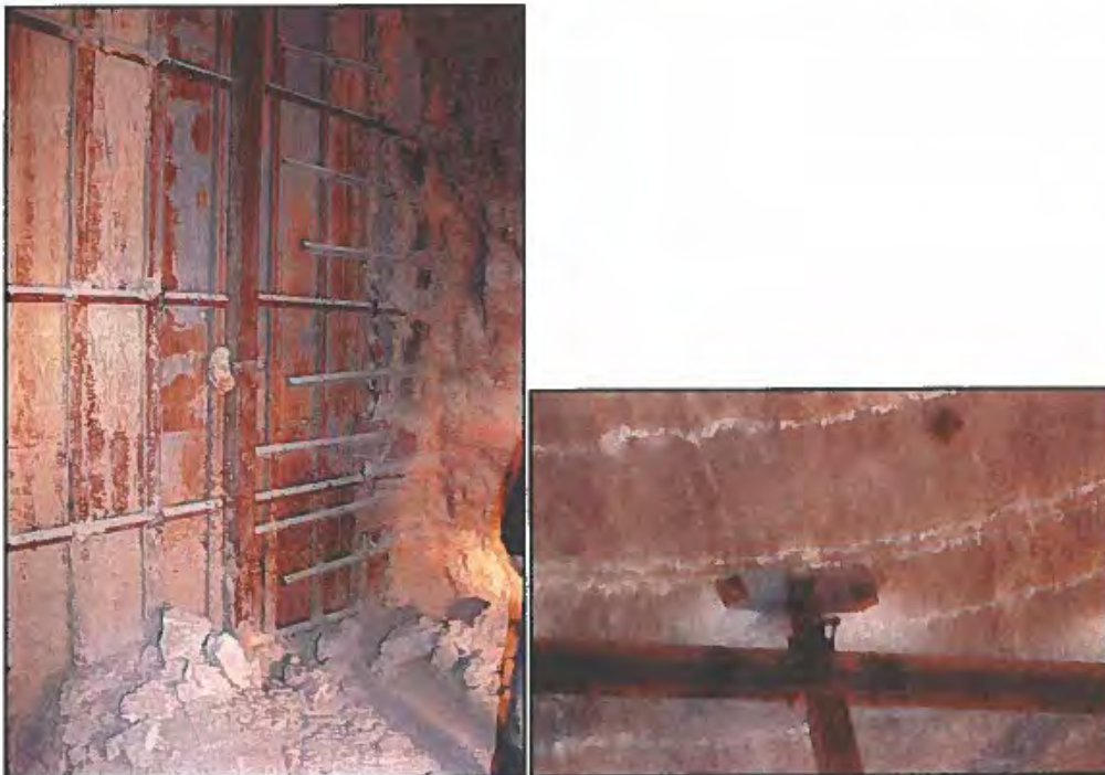
Photographs 11.20 and 11.21 - Stopping fitted to opening using side extensions and ceiling bolts
