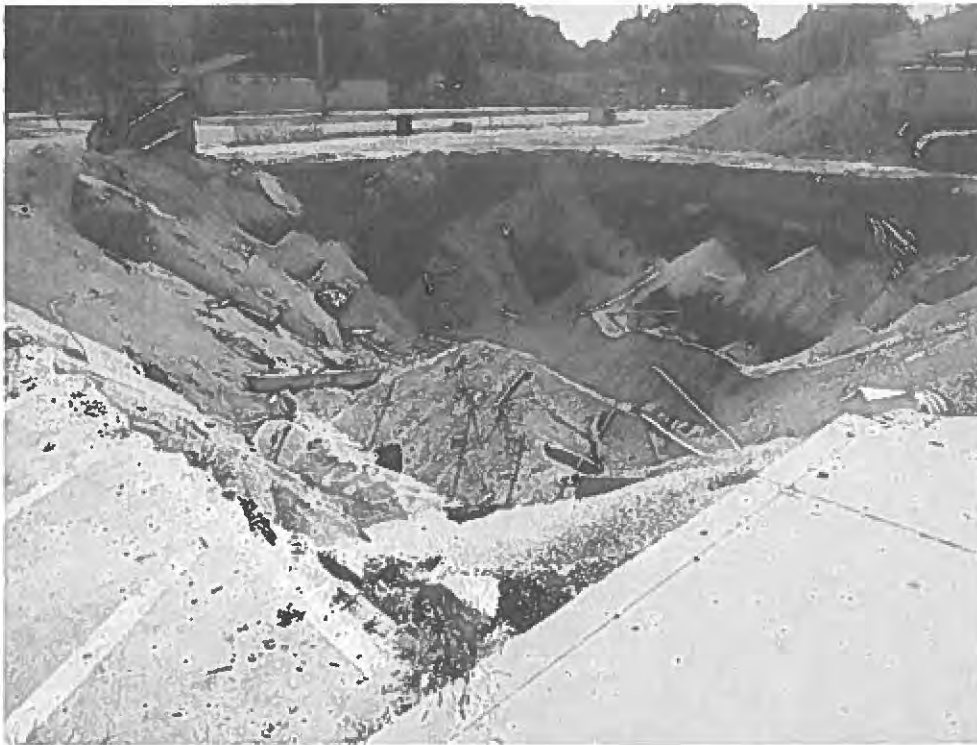
Date: 8/31/2022 Time: 11:18am Direction: NE Photo by: Robert Mileur Exposure #: 013 Comments: Tank field with both UST's removed
