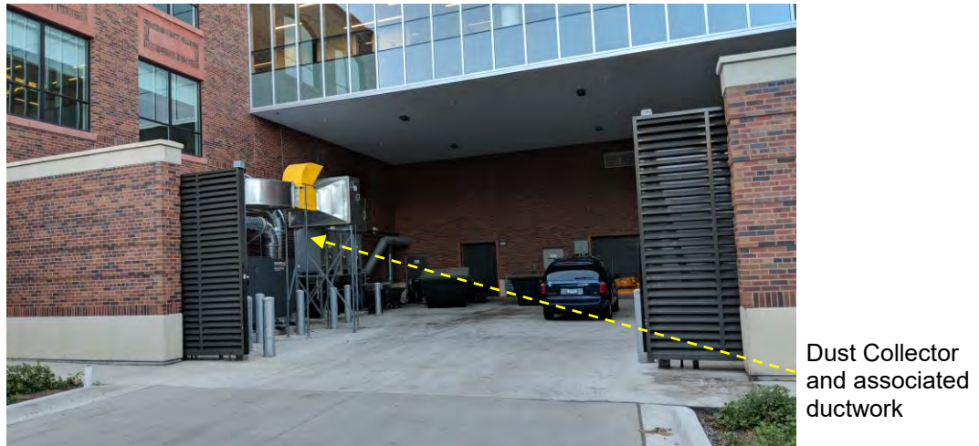
Figure 1. Dust Collector Prior to Construction of Acoustic Barrier – July 25, 2018
