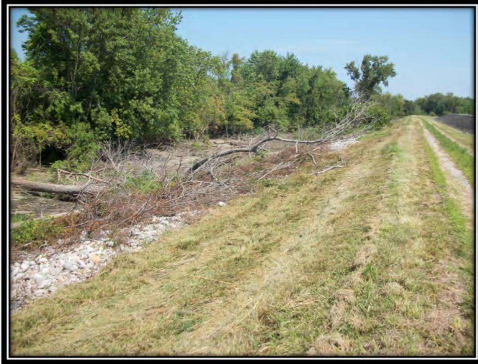
Photo 31 – Fly Ash Pond Embankment (Note Riprap and Felled Tree Debris near Toe)
