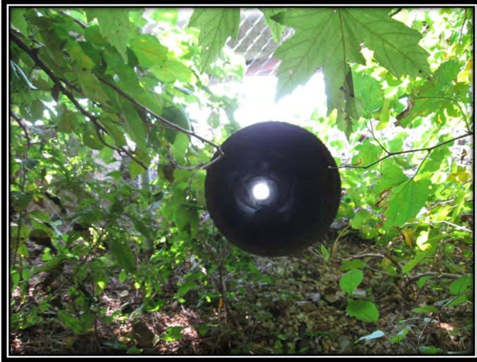
Photo 11 – Emergency Spillway Pipe for the Bottom Ash Pond without any Noticeable Obstructions
