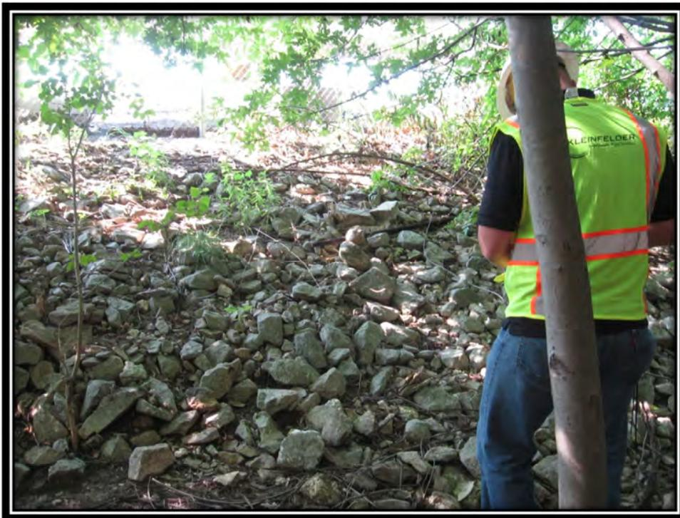
Photo 8 – Riprap on Downstream Slope of Bottom Ash Pond (Typical)
