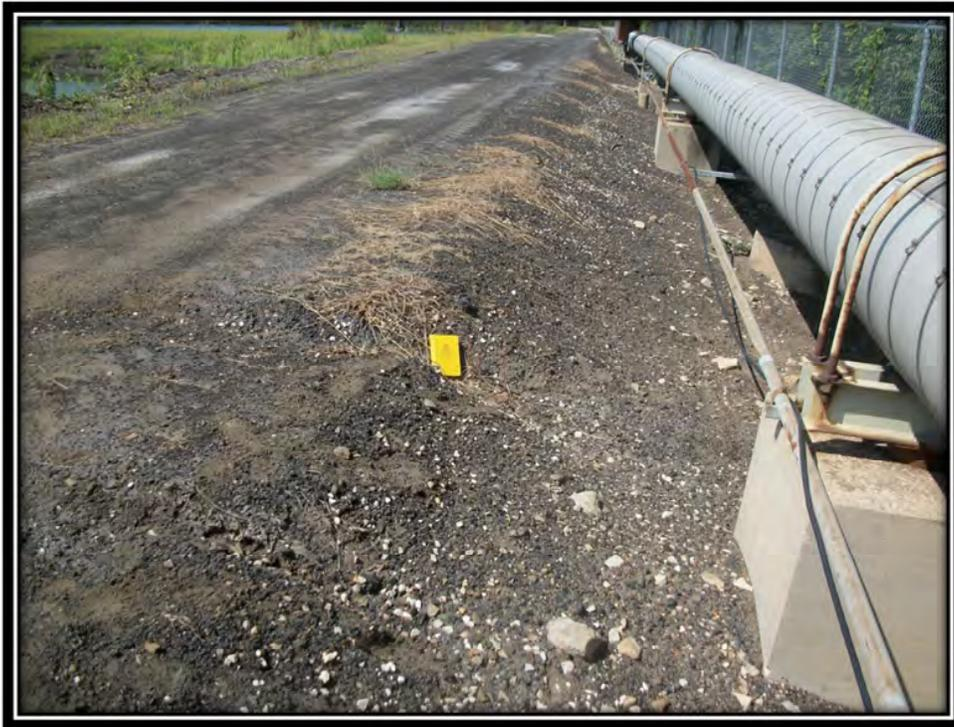
Photo 2 – Minor Surface Erosion of Bottom Ash Pond Crest (Note Typical Crest Condition and Pipeline)
