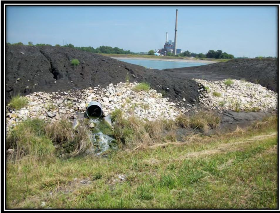
Photo 36 – Fly Ash Pond Culvert Pipe between cells 1 and 4 (Note Emergency Spillway Cut)
