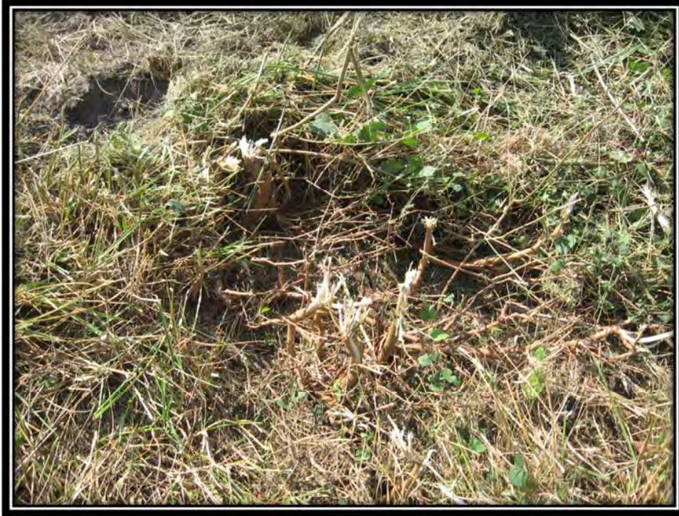
Photo 35 – Mowed Woody Vegetation on Downstream Slope of Fly Ash Pond (Note Intact Root System)
