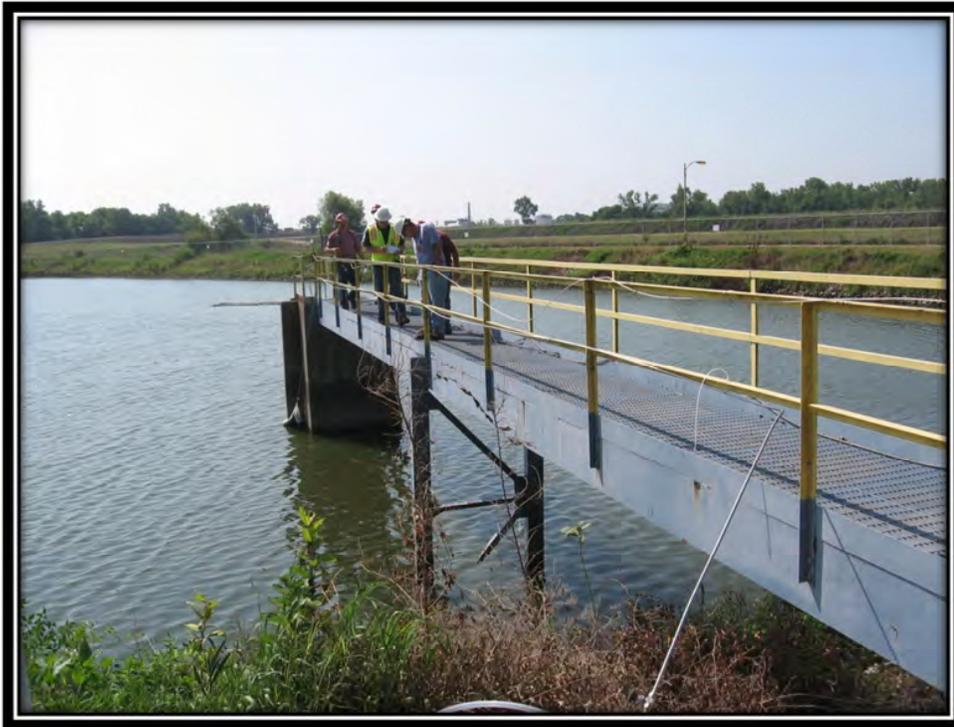
Photo 14 – Outlet Works for the Bottom Ash Pond (Note Broken Support of Walkway)
