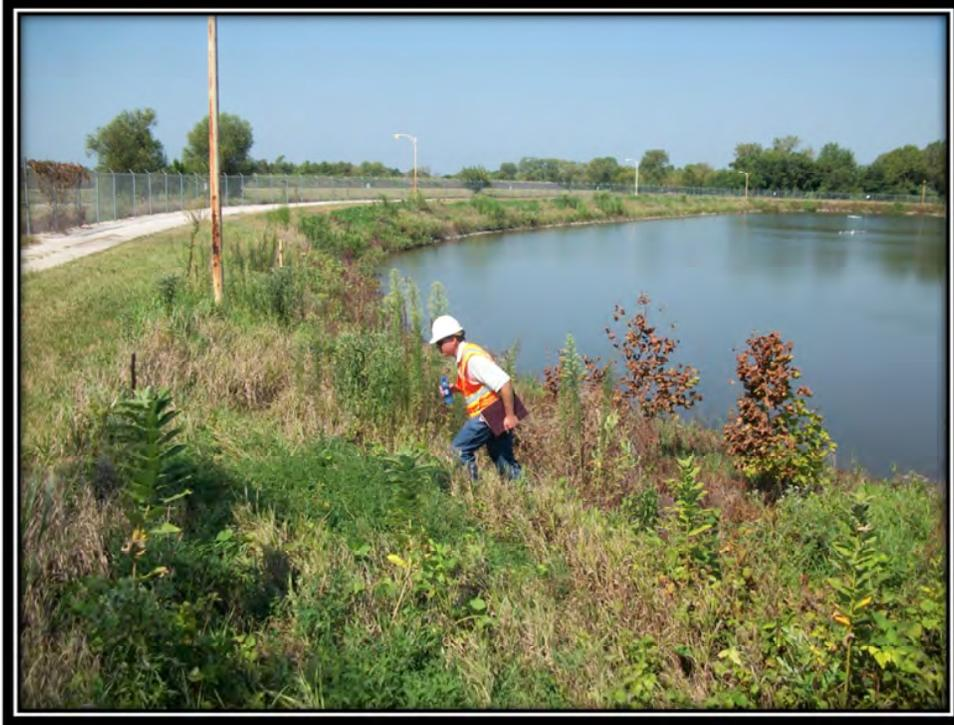
Photo 23 – Upstream Slope of the Bottom Ash Pond (Note Steep Slopes and Light Pole Penetrations)
