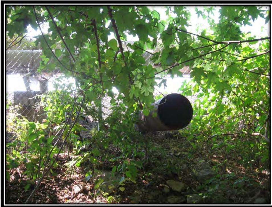
Photo 10 – Emergency Spillway Pipe for the Bottom Ash Pond
