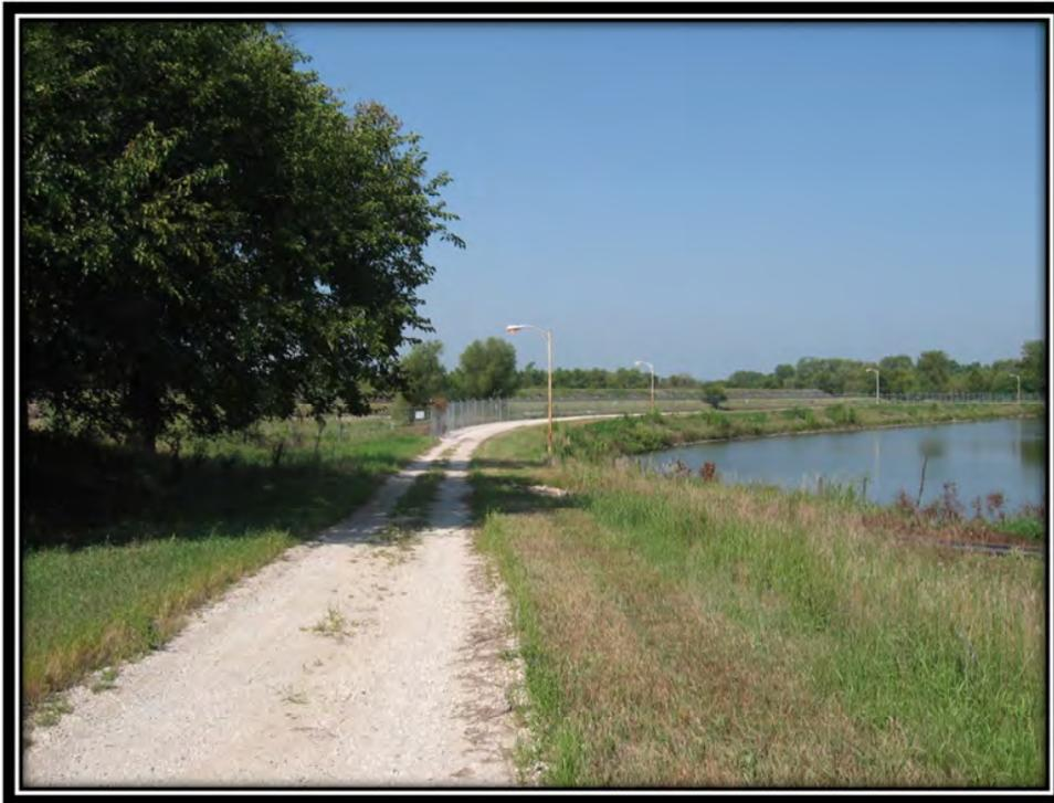
Photo 28 – Typical Crest Condition of the Bottom Ash Pond (Note Light Pole Penetrations in Crest)
