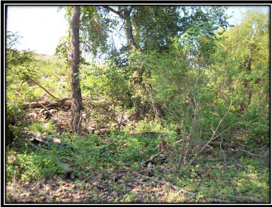
Photo 30 – Vegetation on the Downstream Slope and Toe of the Fly Ash Pond
