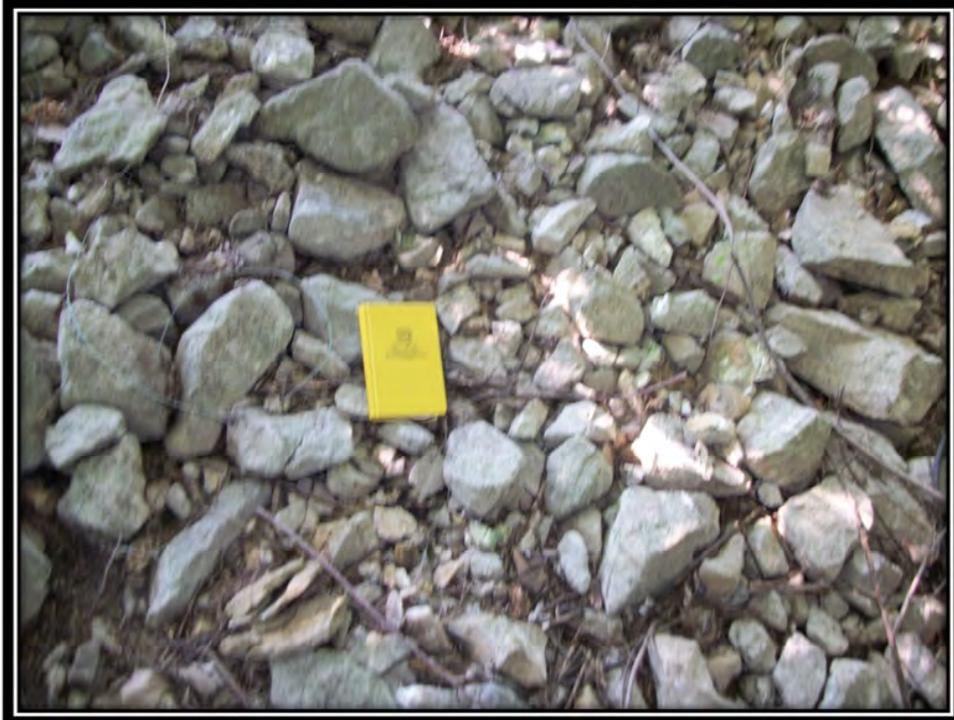
Photo 9 – Undersized Riprap on Downstream Embankment of the Bottom Ash Pond
