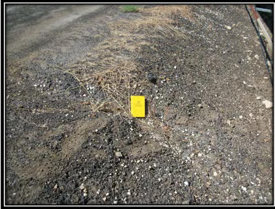
Photo 3 – Minor Surface Erosion of Crest and Downstream Slope of the Bottom Ash Pond (Typical)
