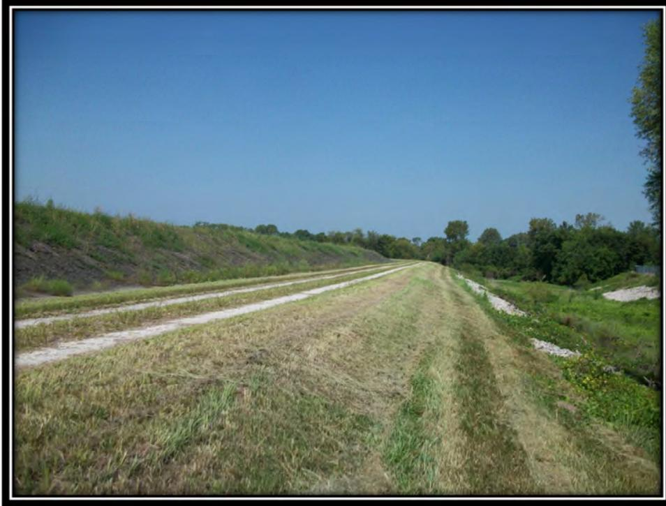
Photo 29 – Typical Embankment of Fly Ash Pond (Note Fly Ash Cell Divider Embankment to Left in Photo)
