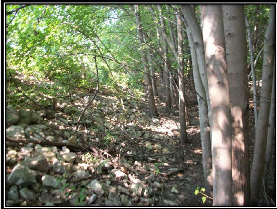
Photo 7 – Riprap and Mature Trees on the Downstream Slope of the Bottom Ash Pond (Typical)
