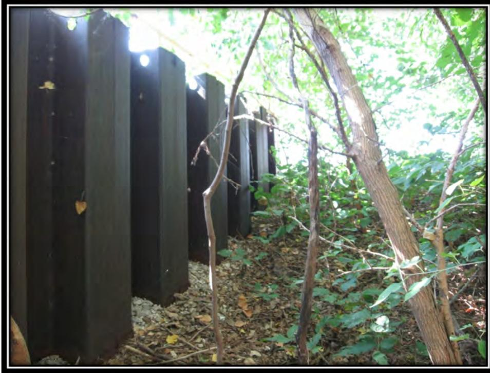
Photo 13 – South Side of the Oil Delivery Sheet Pile Platform (Note Penetration into Embankment)
