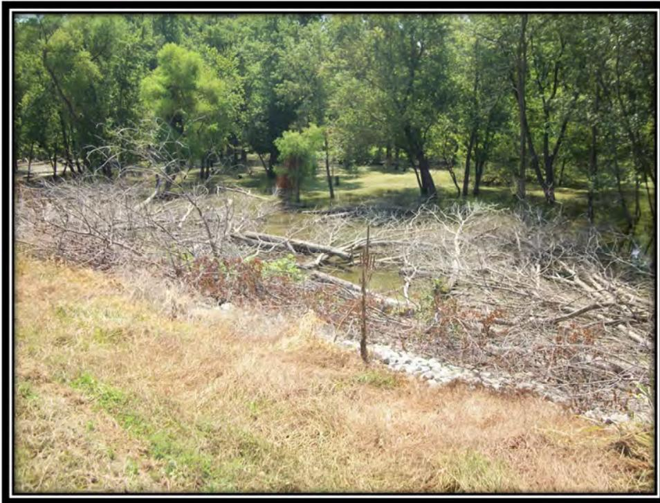
Photo 34 – Flooded Timber and Felled Tree Debris at the Toe of the Fly Ash Pond
