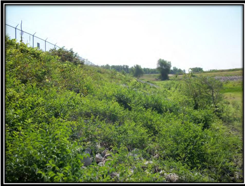
Photo 18 – Vegetated Riprap on the Bottom Ash Pond Southwest Embankment
