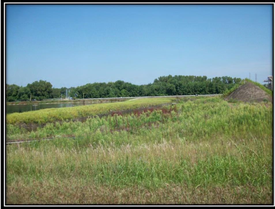
Photo 25 – General Bottom Ash Pond Photograph (Note Bottom Ash Stockpile and Settling Channel)
