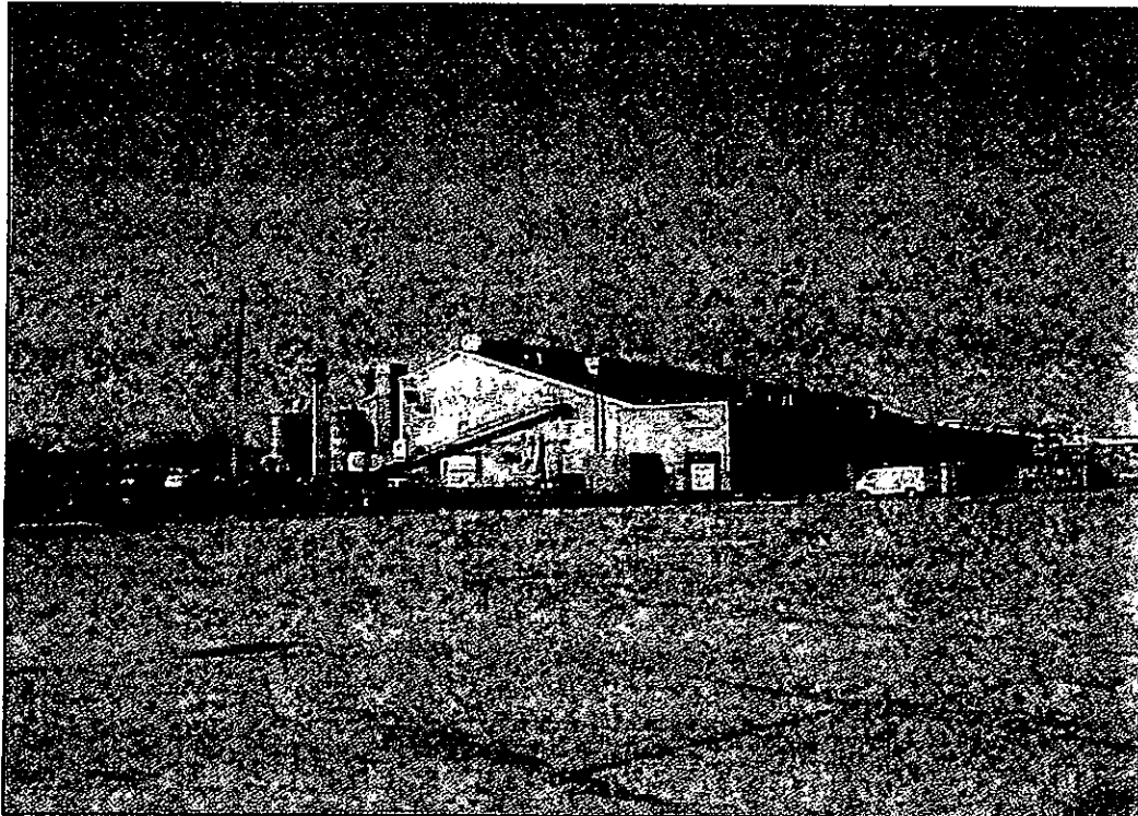
Building 5 as viewed from the northeast.
