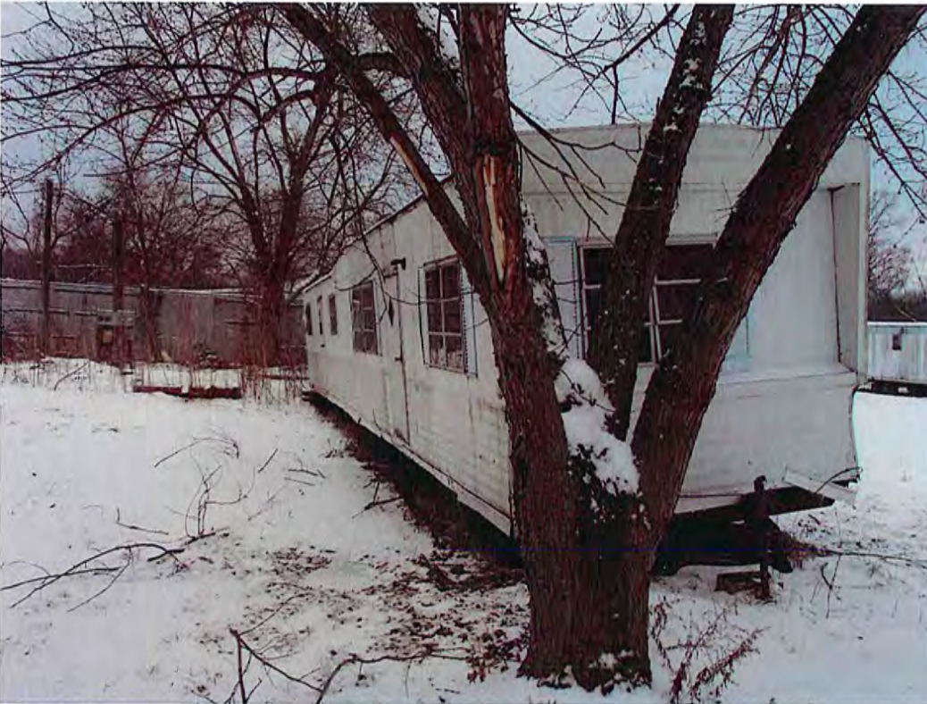
Date: 01/08/2014 Time: 2:23 P.M. Direction: south Photo by: Garrison Gross Exposure #: 002 Comments: waste mobile home (unleveled, no steps and end and front windows open)
