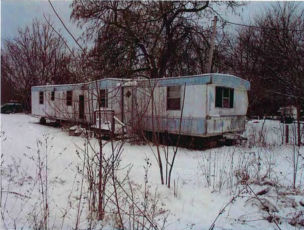
Date: 01/08/2014 Time: 2:23 P.M. Direction: southwest Photo by: Garrison Gross Exposure #: 001 Comments: waste mobile home (overgrown in woody vegetation, missing water tank door and end windows)
