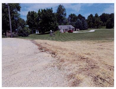
Once the excavation was complete the remaining backfill was delivered and the stockpiled topsoil spread to grade. Left side: edge of former station property; right: Offsite property restored to grade.
