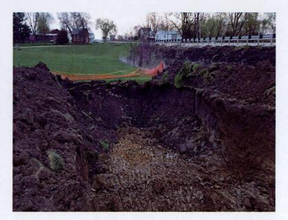
The first phase of soil excavation and removal began on the offsite property east of the subject site. As proposed, the upper 5 feet of topsoil was temporarily stockpiled to provide access to underlying contaminated soils. After the soils were removed and the excavation partially backfilled, the clean topsoil was re-used to bring the site to grade. The surface was later reseeded.
