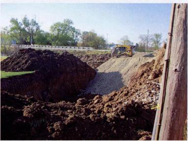
2. The excavation progressed westward along the IDOT right-of-way to the property boundary, then northward onsite. Clean backfill was continuously brought in and graded using a skidsteer to prevent the excavation from becoming too large or unstable.
