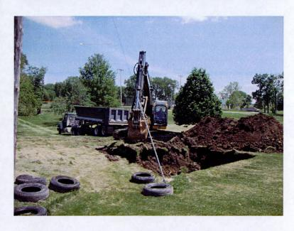
5. The final (third) phase of soil excavation began off-site on the south side of IL Route 24. Surficial soils were temporarily stockpiled while contaminated soils were loaded on semi-trucks for disposal. The topsoil was later used to re-grade and seed the area.
