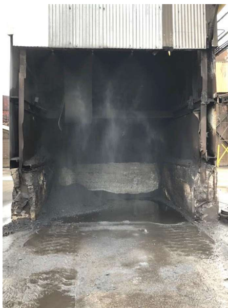
Figure 2 - "3-4 Junction" Building (showing water from overhead sprays)
