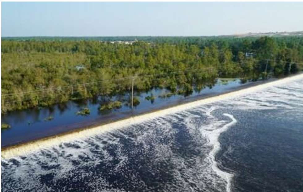
Photograph released by Duke Energy shows flooding from the swollen Cape Fear River overtopping an earthen dike at the L.V. Sutton Power Station near Wilmington, NC. (Washington Post, September 22, 2018)
