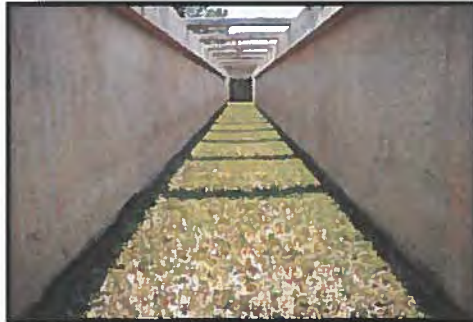
Channel Prepared for Testing
