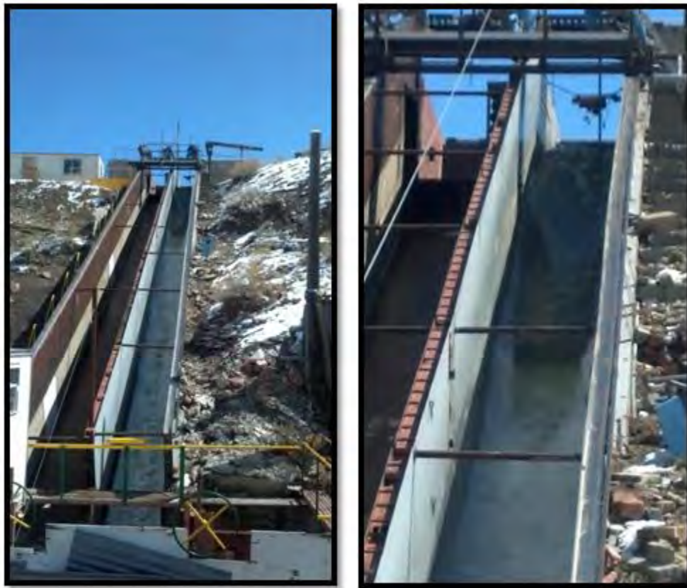
Figure 5 – Steady State Hydraulic Testing of HydroTurf™ at CSU
