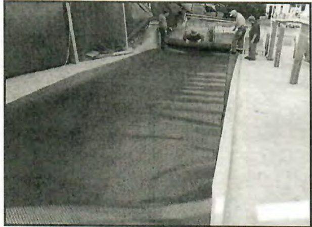
Test Slope Prepared and Liner Installed
