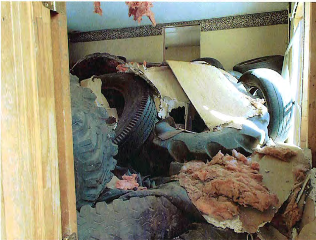
Date: 03/05/2014 Time: 12:58 P.M. Direction: east Photo by: Garrison Gross Exposure #: 010 Comments: used / waste tires stored in mobile home; some were accumulating water through open windows and doors
