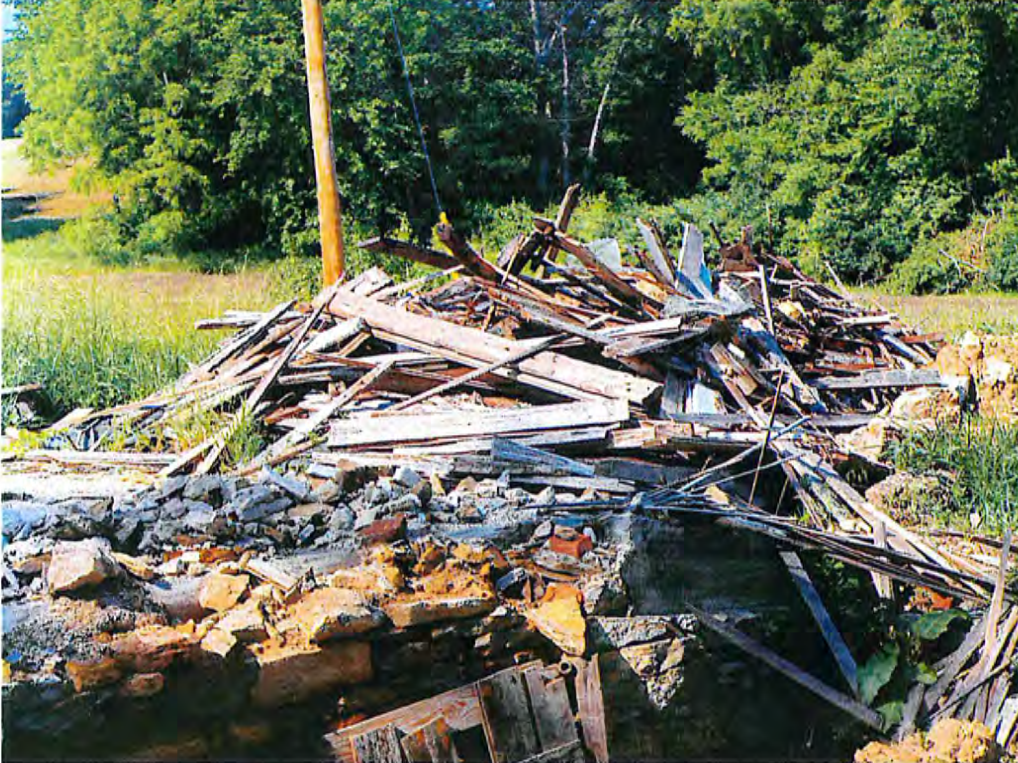
Date: 10/01/2014 Time: 12:32 PM Direction: SE Photo by: Zappa Exposure #: 002 Comments: Another view of the debris and violation that continues.
