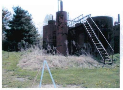
Date: 04/19/2005 Time: 2:31 pm Direction: South Photo by: Rich Johnson Exposure #: 015 Comments: Photo shows the tank battery located along Cotton Hill Road, Note the thin, tall tanks used for separating the water and oil phases of the liquids pumped from the oil production wells. The other tanks hold brine water and oil.
