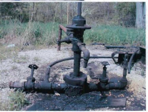
Time: 11:16 am Direction: Northwest Photo by: Rich Johnson Exposure #: 004 Comments: Photo shows Galloway #3 production well located in the southwest region of the Galloway lease. Note the wellhead and the associated pipes and valves.
