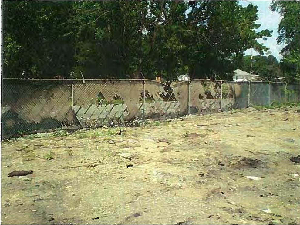
Date: 5-8-12 Time: 11:41am Direction: NW Photo by: P. Fatka Exposure #: 005 Comments: Fire damaged fence.
