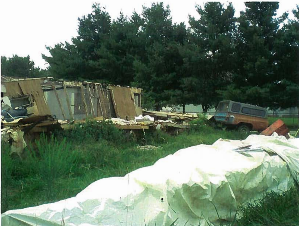
Date: August 9, 2010 Time: 10:56 Direction: SE Photo by: S. Townsend Exposure #: 008 Comments: Demolished mobile home wastes.
