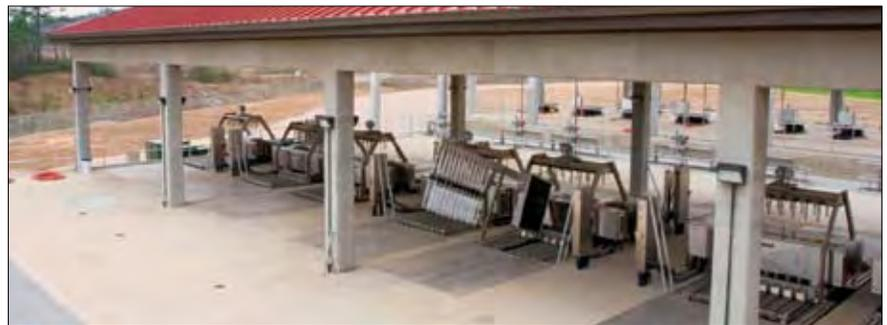
*The eight TrojanUV4000Plus™ reactors used to disinfect 600 MGD (94,680 m<sup>3</sup>/hr) at this large wastewater treatment facility require a footprint measuring only 80' x 120' (24 x 36 m) – a fraction of the space needed for chlorine disinfection.*
