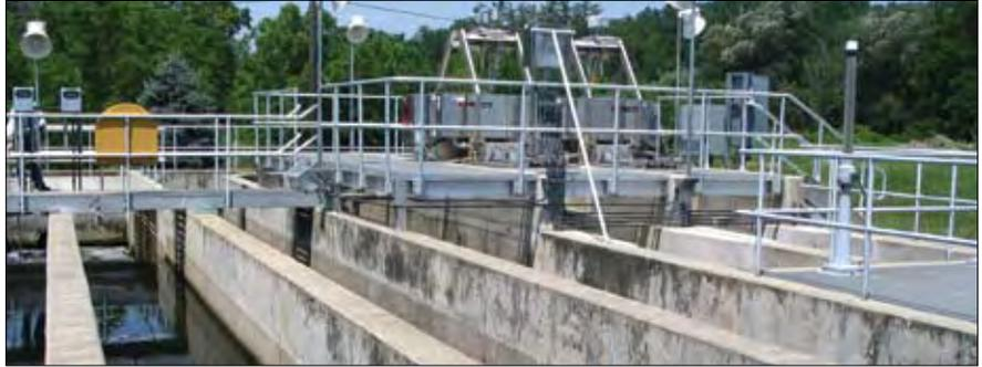
*In this retrofit installation, each reactor was installed in one pass of the existing chlorine contact basin with only minor modifications to the channels. This allows the majority of the basin to be used for storage, by-pass or emergency back-up.*
