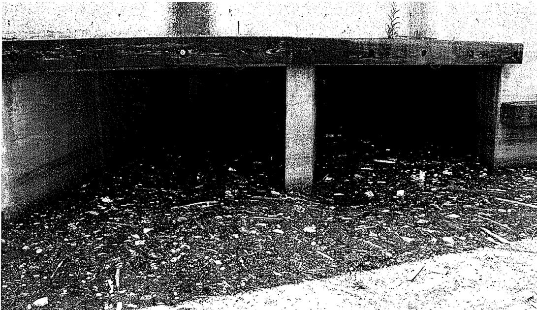
*Figure 3: Floatable Debris Collected at RAPS Following a CSO Event*
