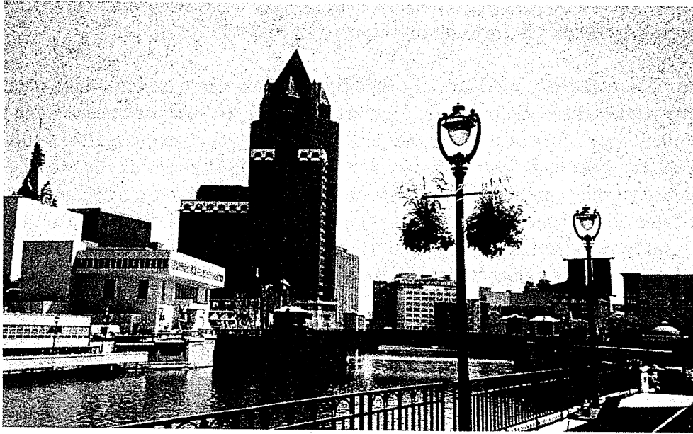
Figure 8.2 Milwaukee River in Downtown Milwaukee (WI). The river is constricted by downtown development, is maintained as a navigable channel and has poor habitat and reeration. Relatively good water quality is provided by pumping lake water into it at a point upstream of the downtown.
