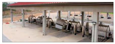
The eight TrojanUV4000Plus<sup>™</sup> reactors used to disinfect 600 MGD (94,680 m<sup>3</sup>/hr) at this large wastewater treatment facility require a footprint measuring only 80' x 120' (24 x 36 m) – a fraction of the space needed for chlorine disinfection.
