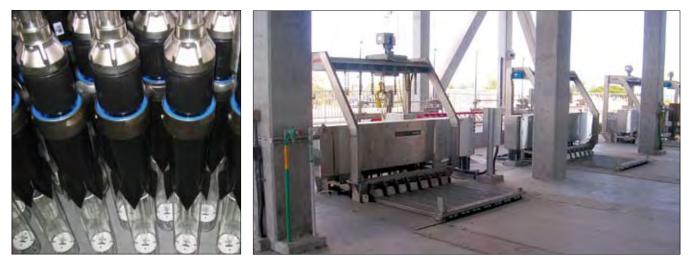
The TrojanUV4000Plus<sup>™</sup> has been optimized for disinfection of low quality wastewater using high intensity lamps, and vortex mixers (left) to increase flow turbulence around the lamps. Trojan's UV technology allowed the City of Honolulu, Hawaii to disinfect primary effluent at their Sand Island treatment facility (right), and thereby save hundreds of millions of dollars that would have been required to build secondary treatment facilities.
