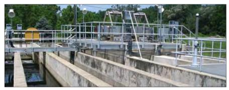
In this retrofit installation, each reactor was installed in one pass of the existing chlorine contact basin with only minor modifications to the channels. This allows the majority of the basin to be used for storage, by-pass or emergency back-up.
