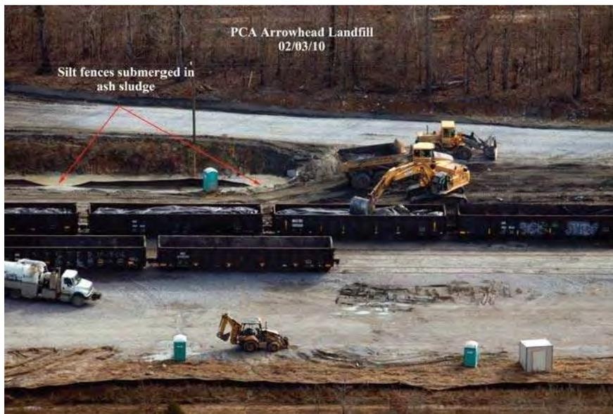
**Figure 6: Fly ash unloading from rail cars at Arrowhead Landfill, AL**
