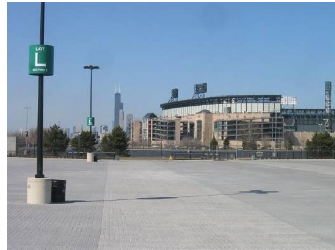
Permeable pavement at White Sox Park
