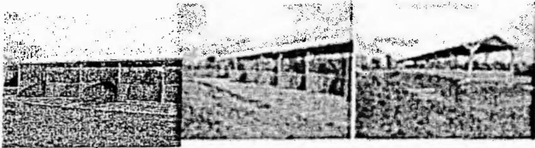
Dead cattle from the cattle barns are composted in the composting barn. Due to the roof structure, animals and composting material is completely protected from rainwater, eliminating possible runoff.
