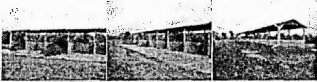
Dead cattle from the cattle barns are composted in the composting barn. Due to the roof structure, animals and composting material is completely protected from rainwater, eliminating possible runoff.
