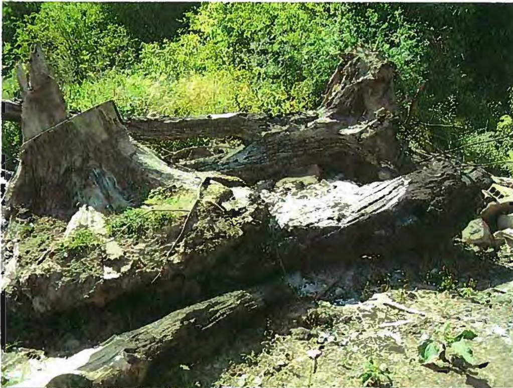
Date:05/17/12 Time: 2:30 PM Direction: NW Photo by: Zappa Exposure #: 001 Comments: One view of area where open burning of demolition took place.
