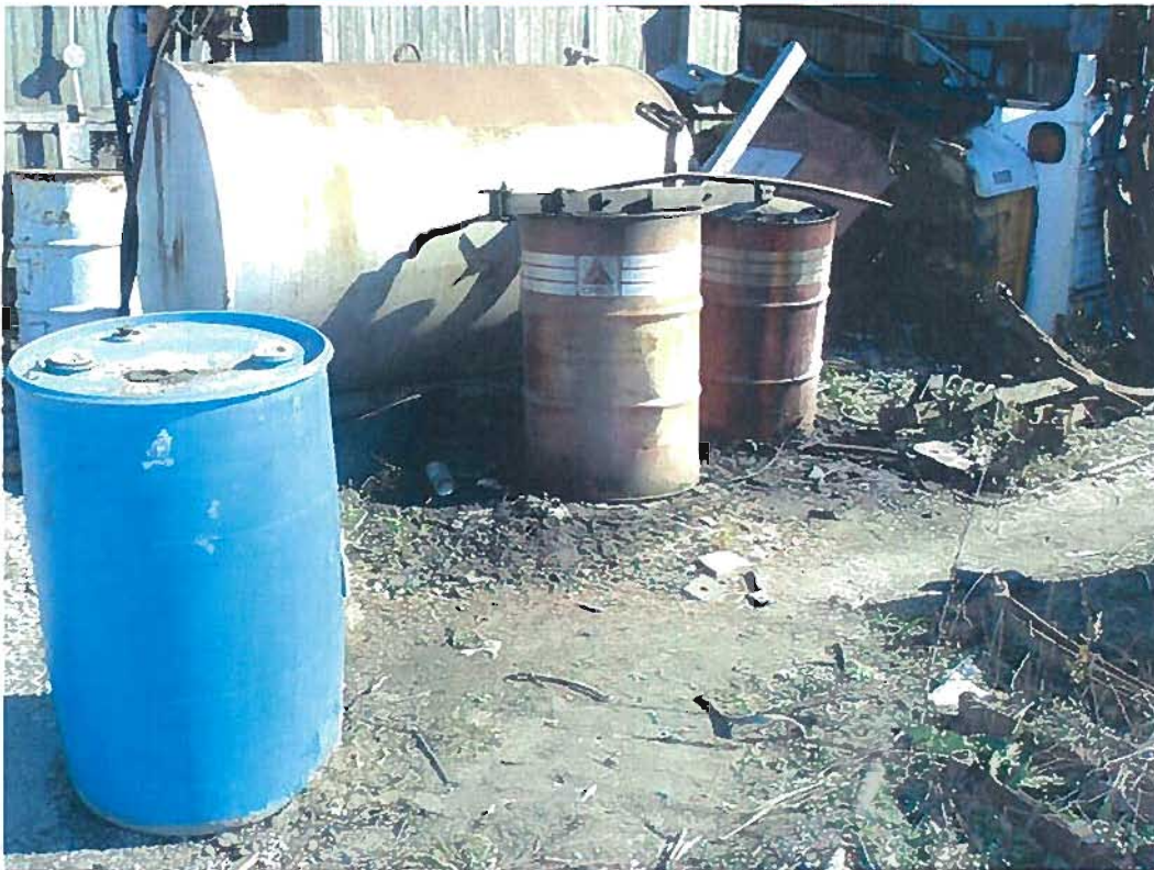
Date: 10/25/2011 Time: 2:20 P.M. Direction: southeast Photo by: S. Williams Exposure #: 022 Comments: apparent leak in area of two metal drums
