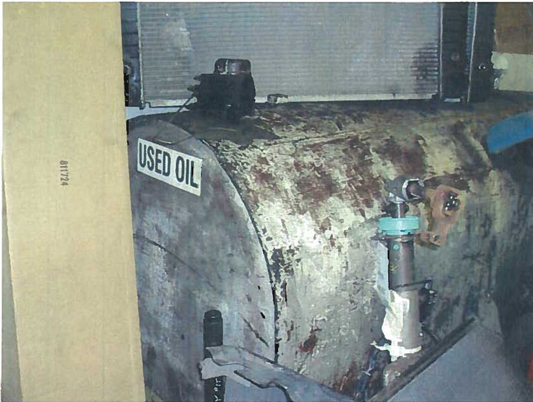
Date: 10/25/2011 Time: 12:49 P.M. Direction: northwest Photo by: S. Williams Exposure #: 015 Comments: used oil tank is labeled
