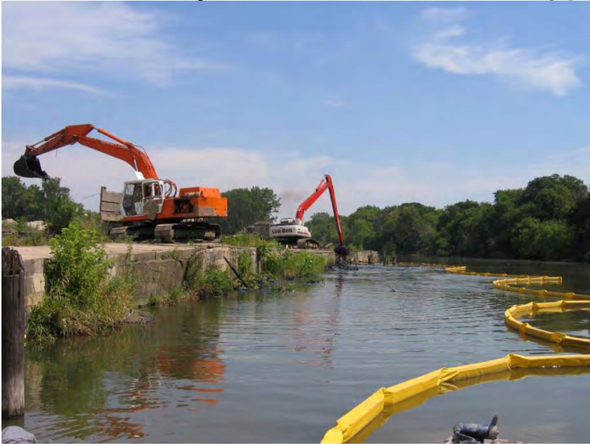
Dredging operations to remove concrete wall and widen and deepen the river in preparation of reshaping shoreline and installation of docks.
