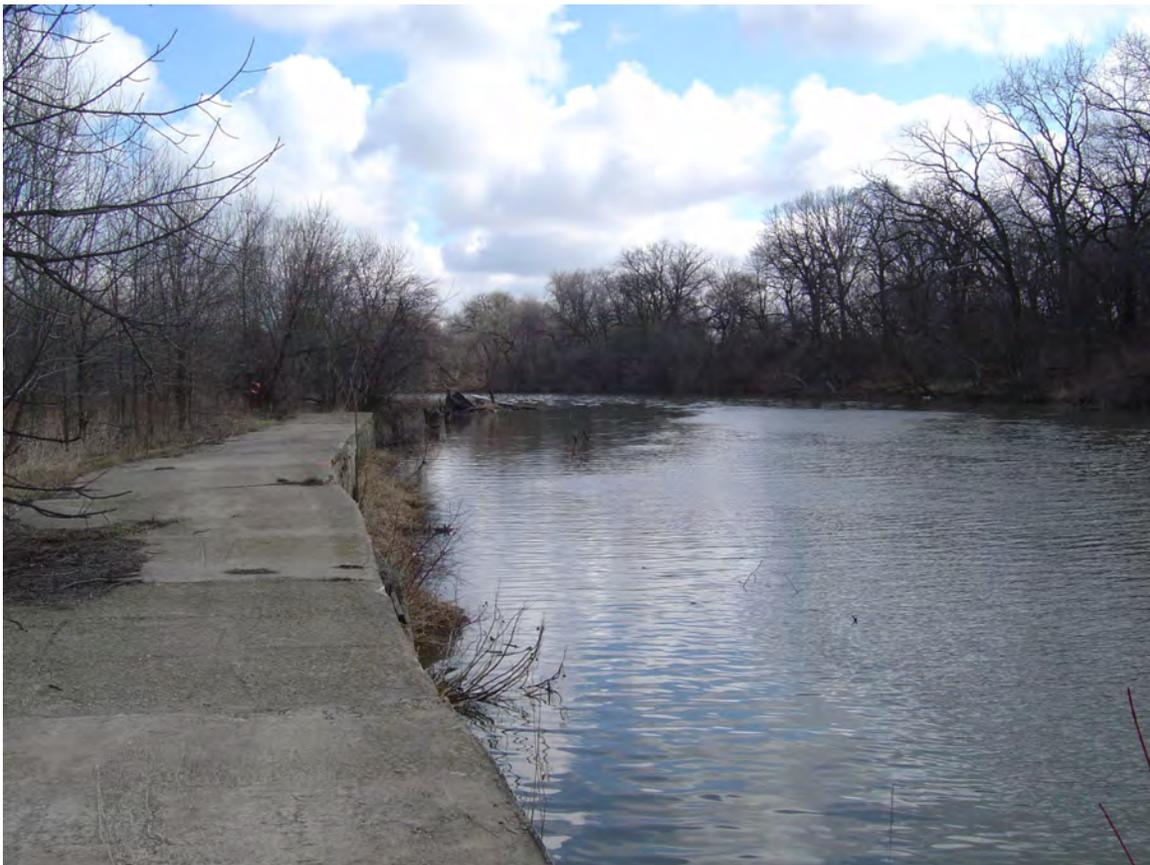
Shoreline in 2004 before work was started. Remnants of the old Marina and 800' concrete wall, and broken riprap comprises most of the river's edge
