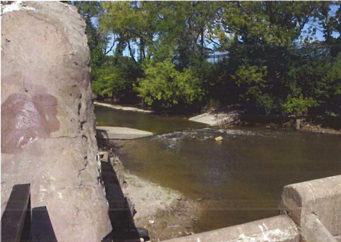
Figure 5.5 – Submerged concrete walkway immediately upstream of the North Branch Dam.
