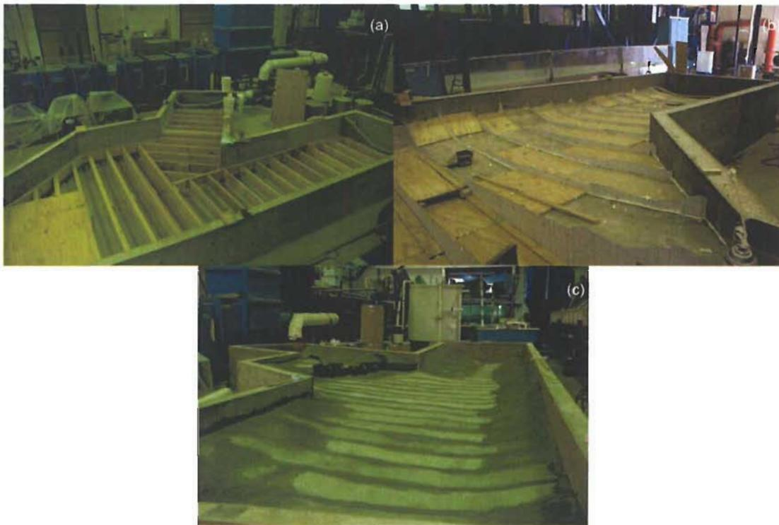
**Figure 4.2 – Photograph of the physical model construction.**
