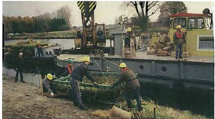
*Placement of individual vegetated revetment modules is easily accomplished when using a crane and requires little manual labor.*
