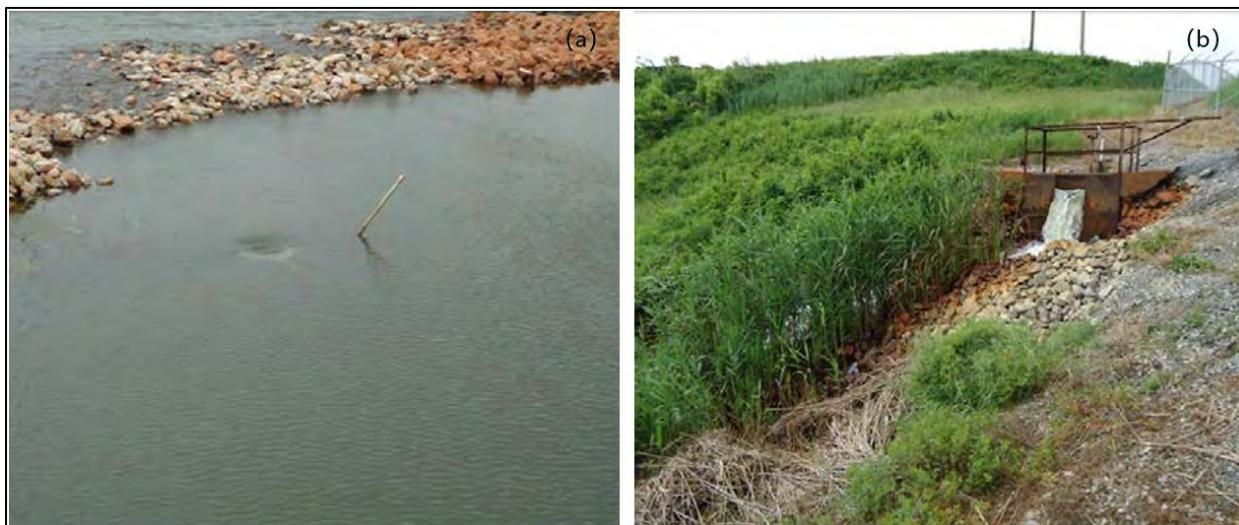
**Figure 3.4 2011 Photographs of Pond 4 – (a) Intake from Pond 4 to Outlet Structure (pipe submerged); (b) Outlet Structure from Pond 4.** Source: Kleinfelder, 2013.
