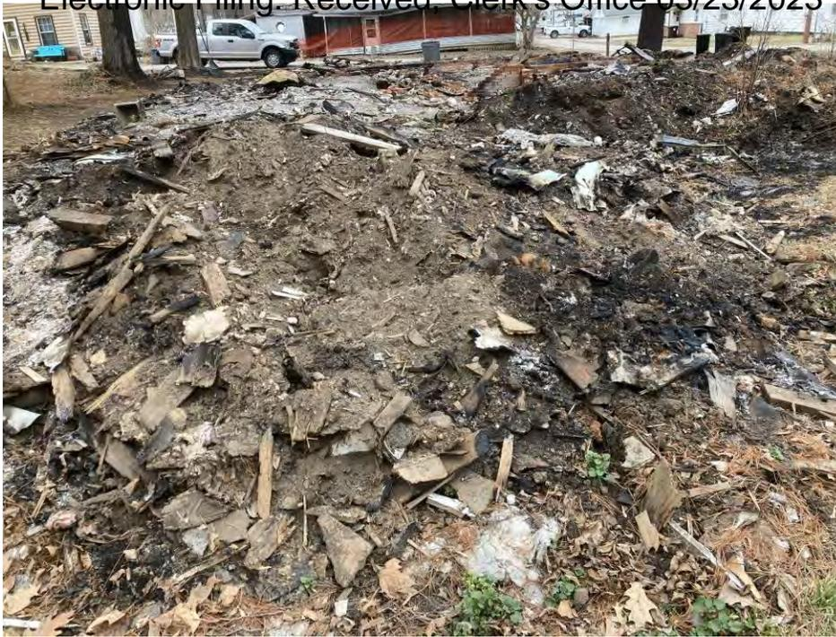
Demolition waste, along the outside of the foundation, illustrates that the residence was razed prior to the burning of the structure.
