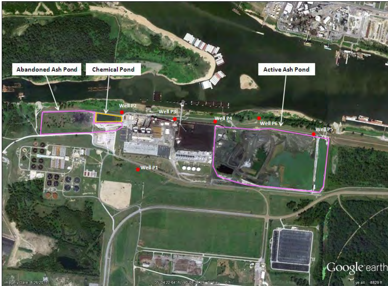
Figure 2-1: Groundwater wells at Allen Fossil Plant (approximate locations)
