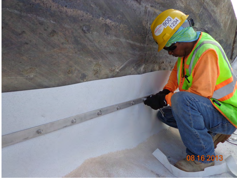
Batten strip connection along the outfall (looking south)
