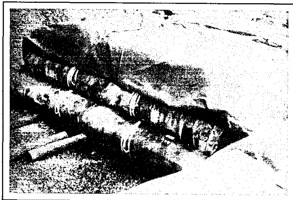
Figure 4.5(b) - Photograph of Temporary Storage of GCLs at Project Site
