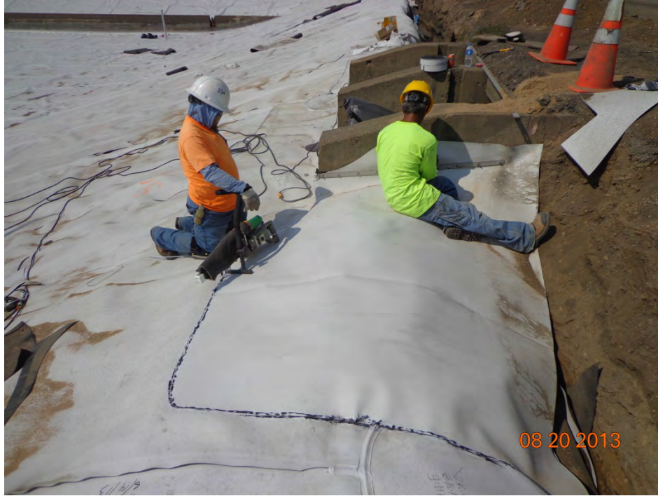
Second layer of geomembrane placed over clean, backfill sand (looking north)
