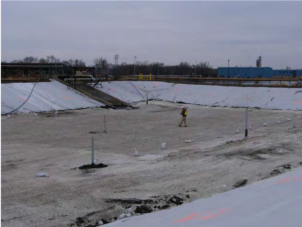
View of the bypass basin during the leak location survey.
