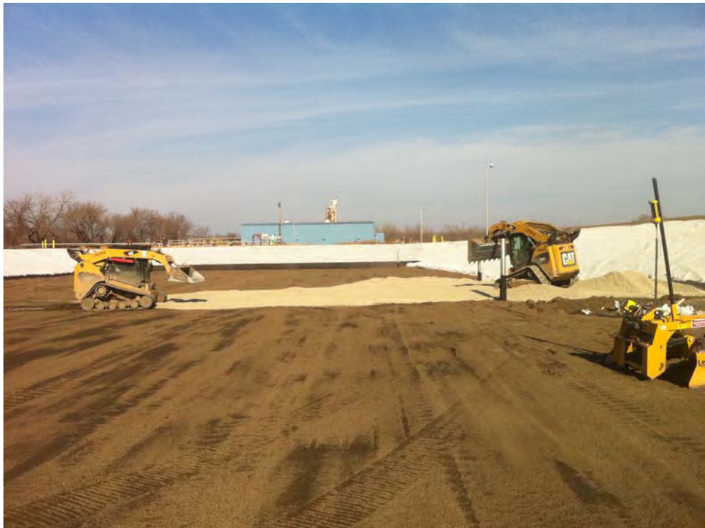
View of finished cushion layer and beginning of warning layer.
