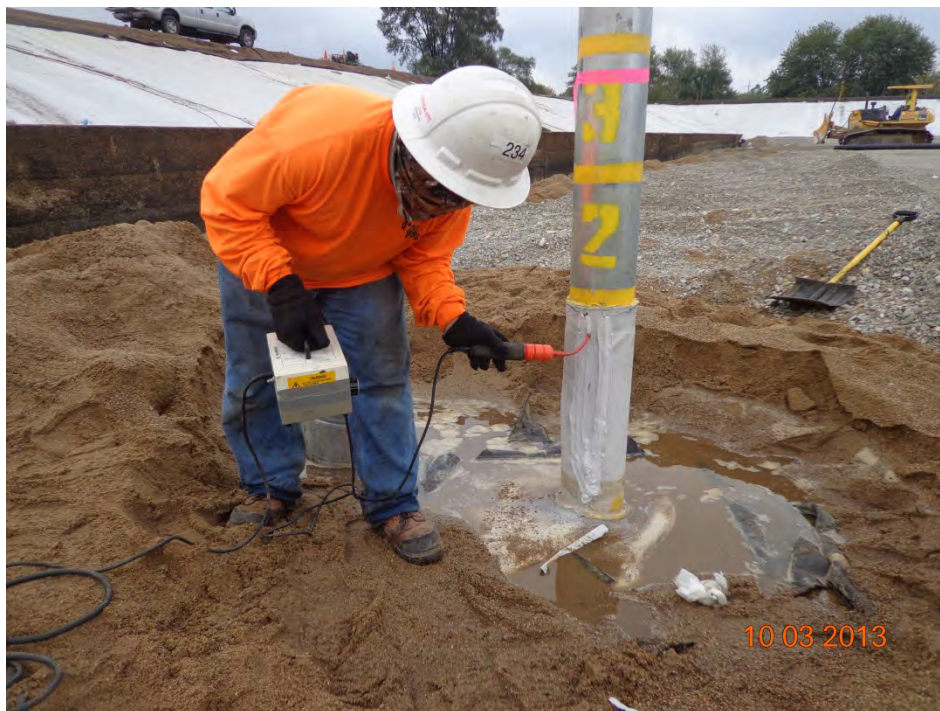
Spark testing the new repairs (looking northeast)
