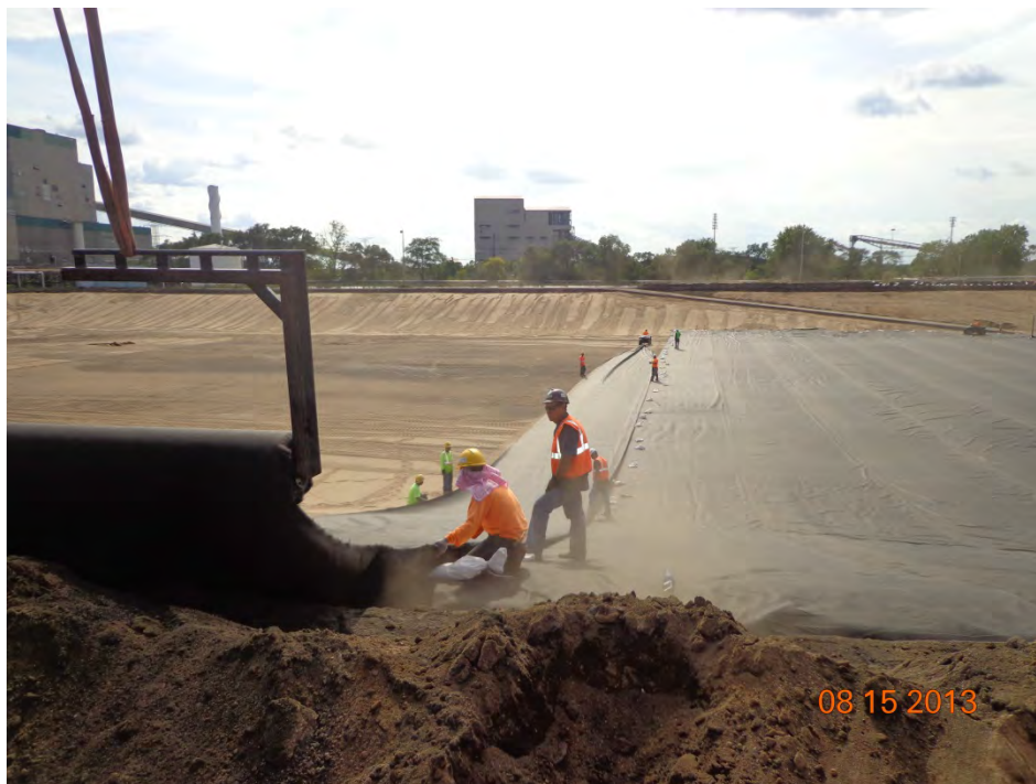
Deployment of geotextile (looking west)
