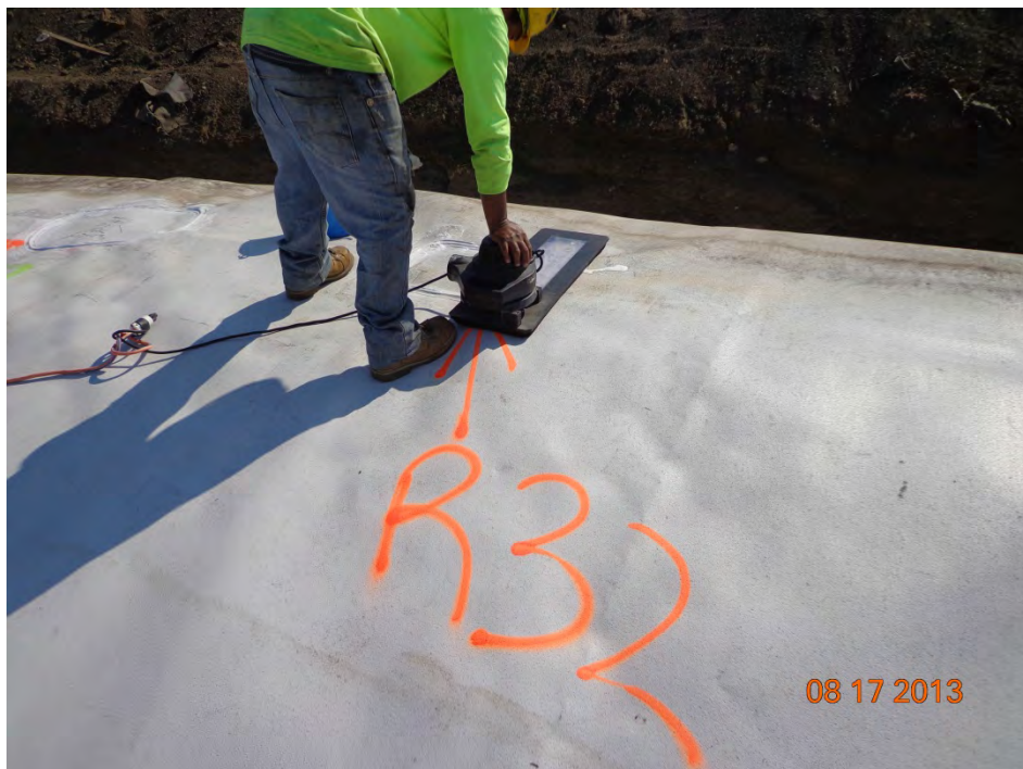
Vacuum testing a repair location
