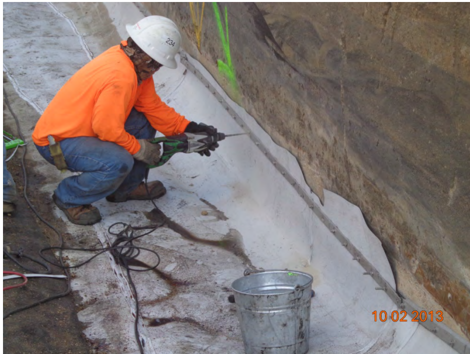
Repairs on batten strip
