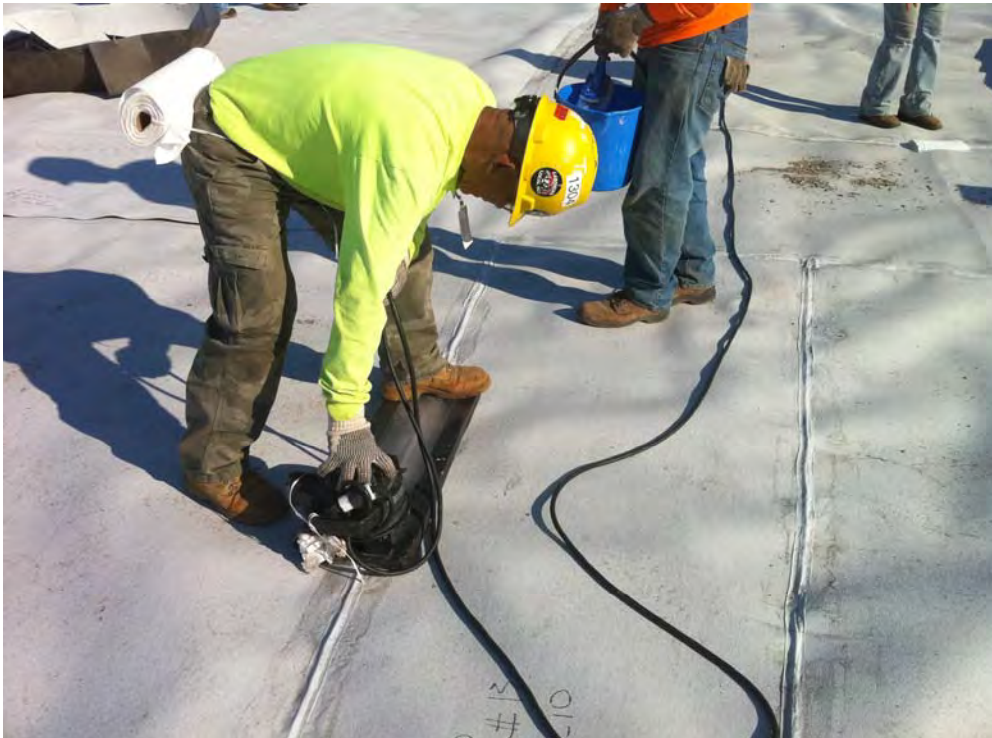
View of extrusion seaming vacuum testing.
