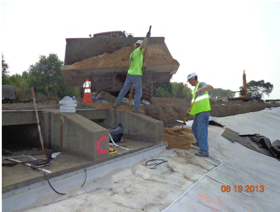
Placing sand around overflow structure (looking southeast)
