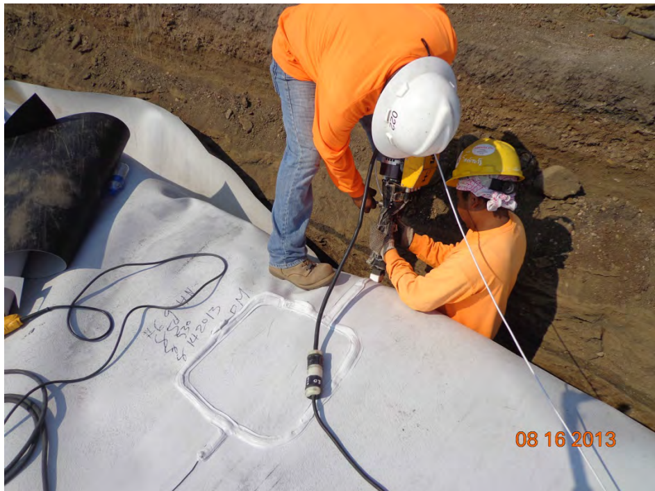
Extrusion weld on a repair location
