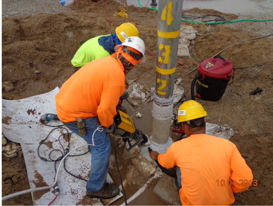
Last of the riser poles being fixed
