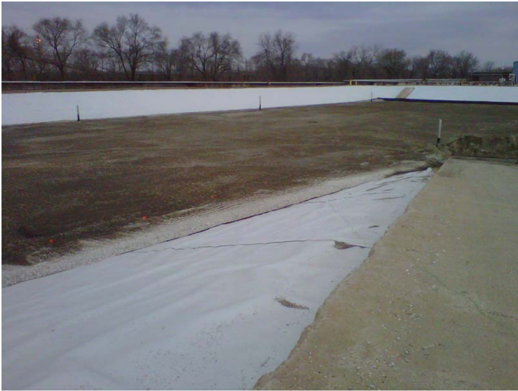
View Looking Northwest Along Ramp.
