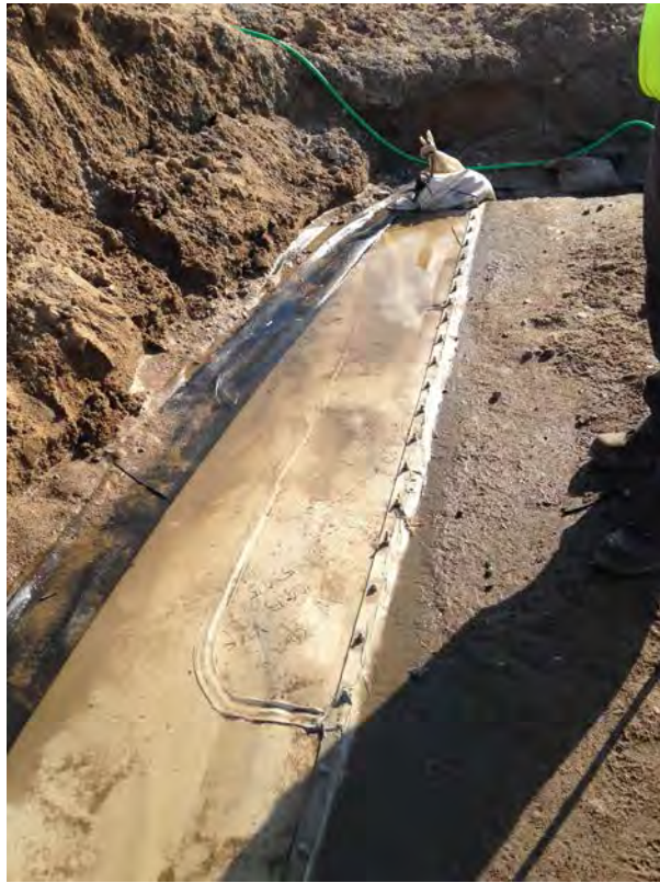
Damaged connection to batten strip on north side of weir wall, facing southwest
