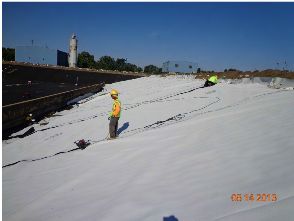
Seaming of the geomembrane panels (looking west)
