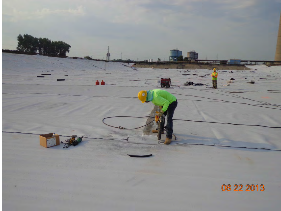
Extrusion welding a geomembrane repair in progress (looking south)
