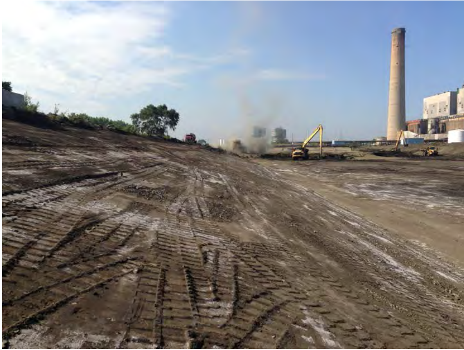
South-facing view of eastern slope, Poz-O-Pac and transition in good condition, some ash remains that will be removed
