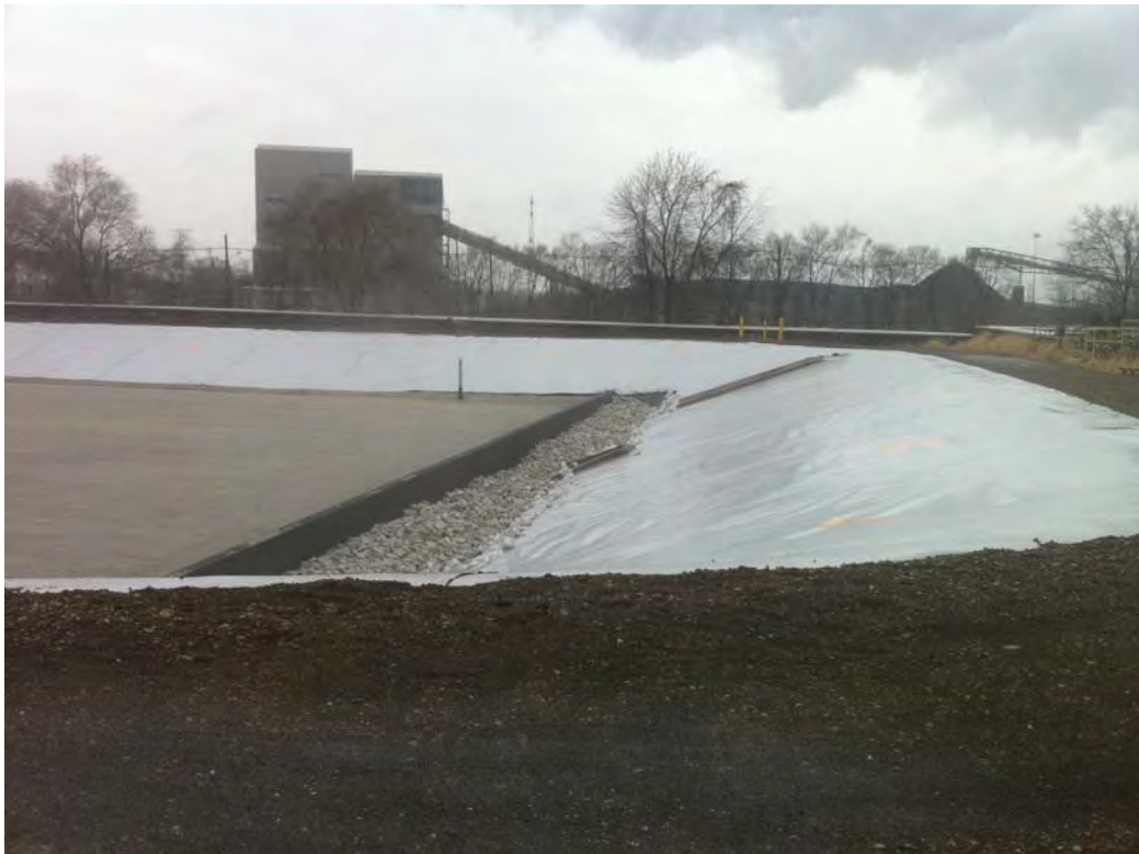
View of finished rip rap north of weir wall.
