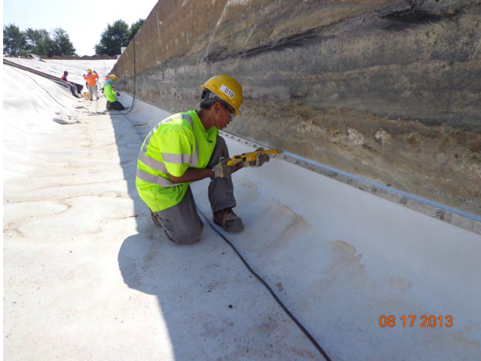
Caulking liner termination on the weir wall (looking east)
