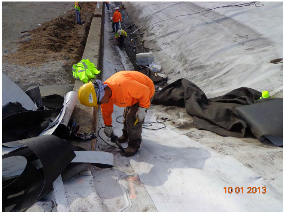
Batten strip repairs underway (looking west)
