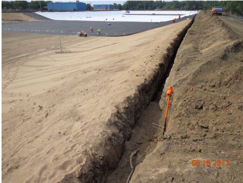
Extent of geotextile and HDPE deployment completed (looking north)
