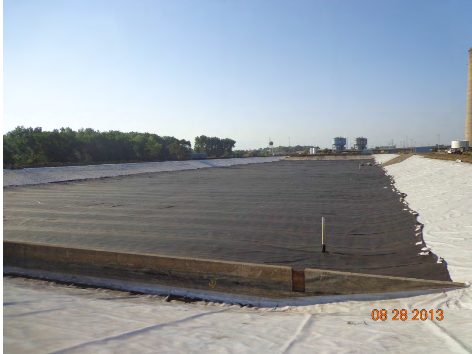
Extent of the completed geosynthetics (looking southeast)
