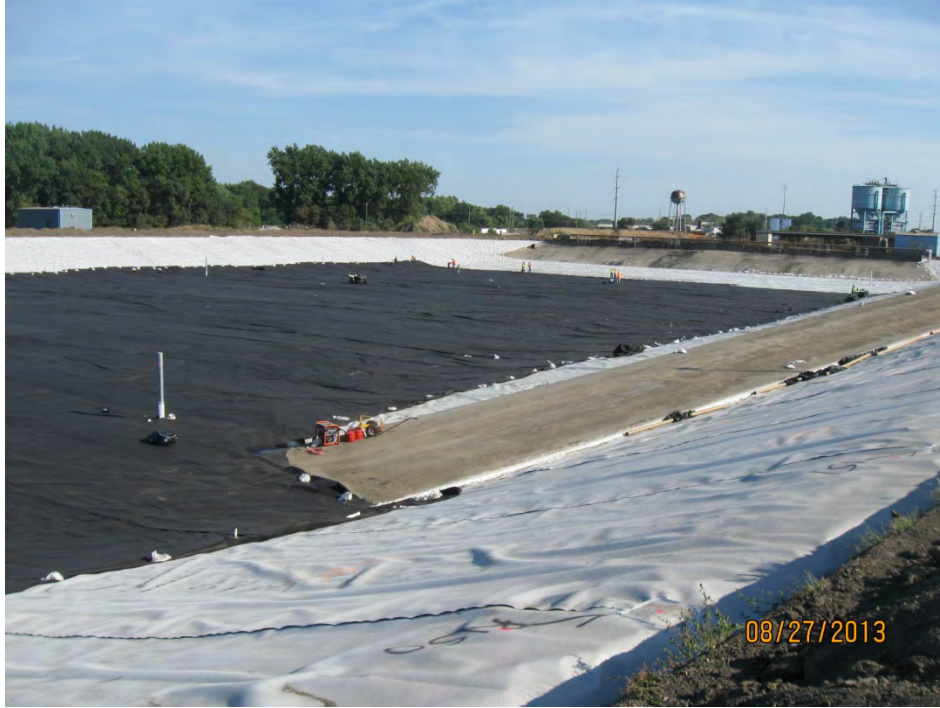
Extent of upper nonwoven geotextile installation completed to date (looking southeast)
