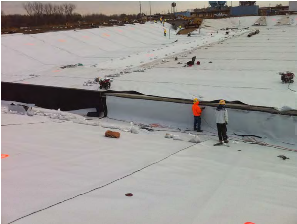
View of liner being attached to weir wall HDPE weld strip.
