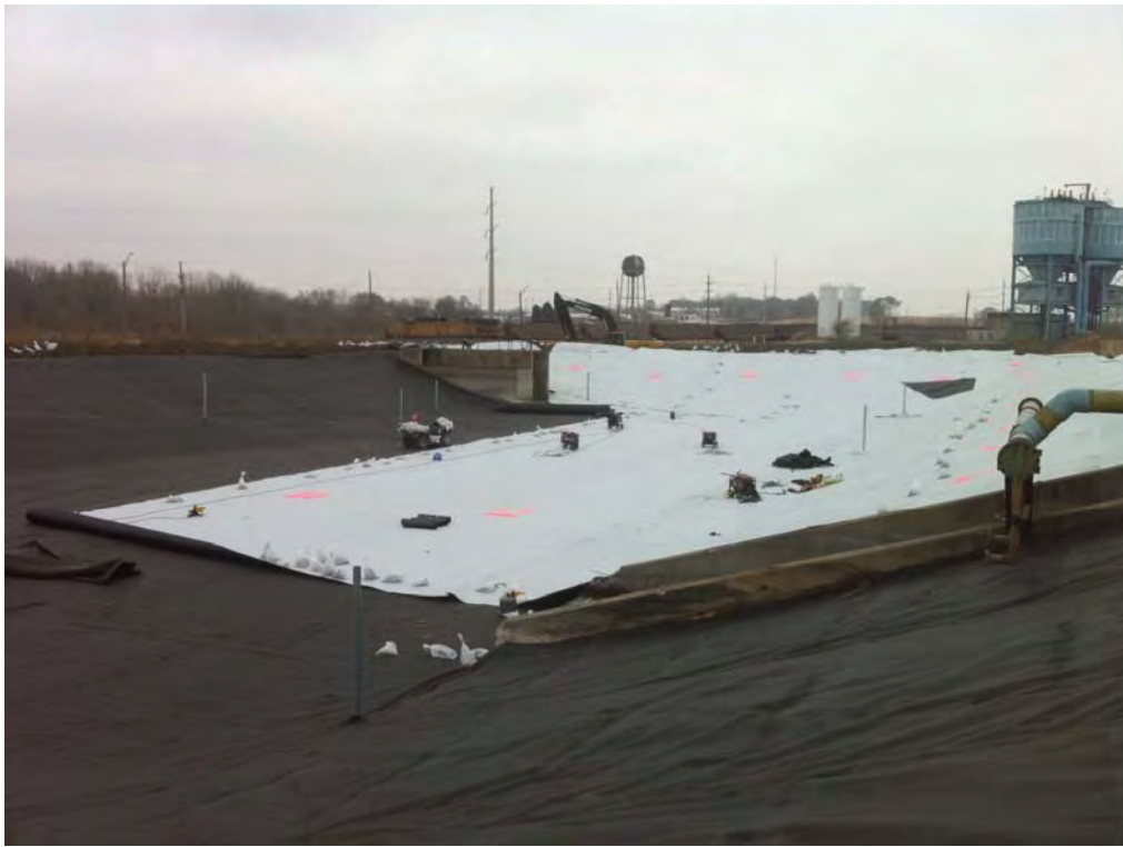
View of 16 oz geotextile in place and HDPE liner being placed.
