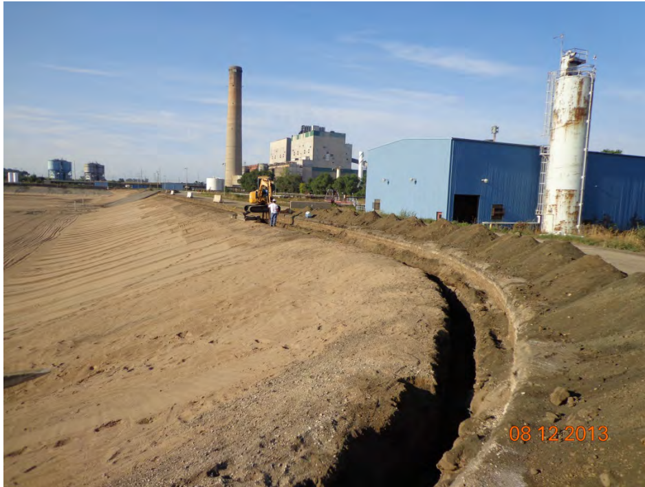
Terra Crew digging the anchor trench around the basin (looking southwest).
