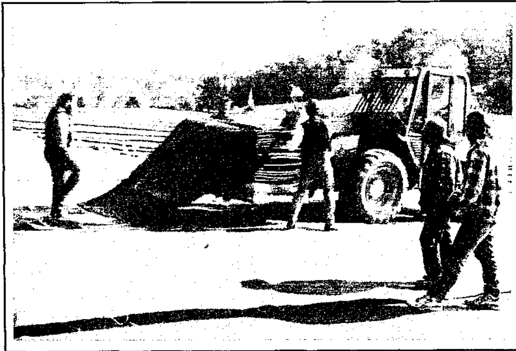
Figure 3.16 - Photographs Showing the Unrolling (Upper) and Unfolding (Lower) of Geomembranes
