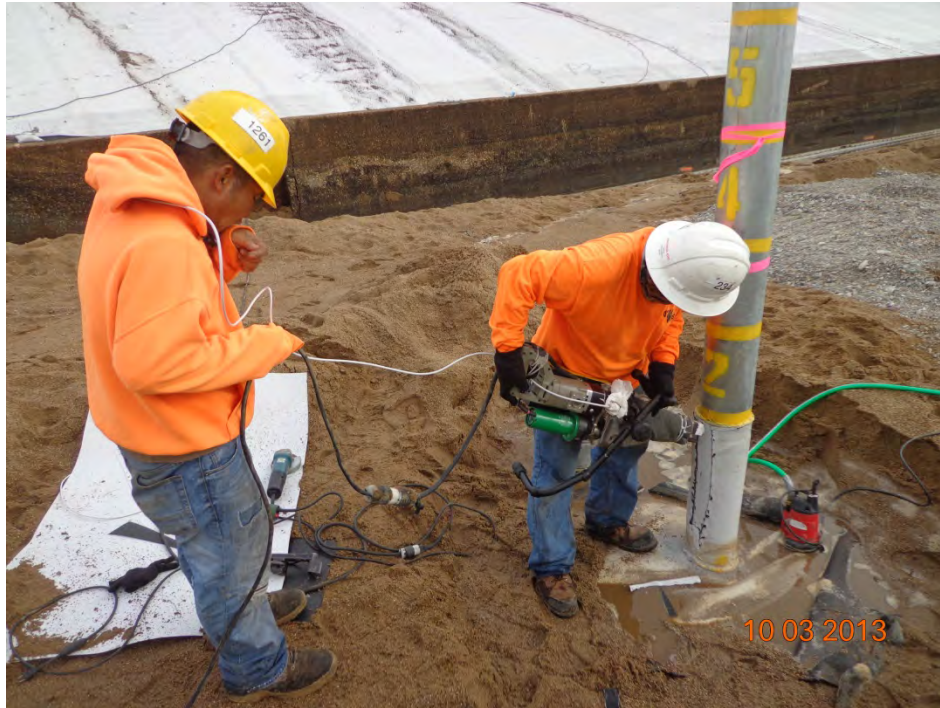
One of the riser pole geomembrane boots being fixed (looking north)
