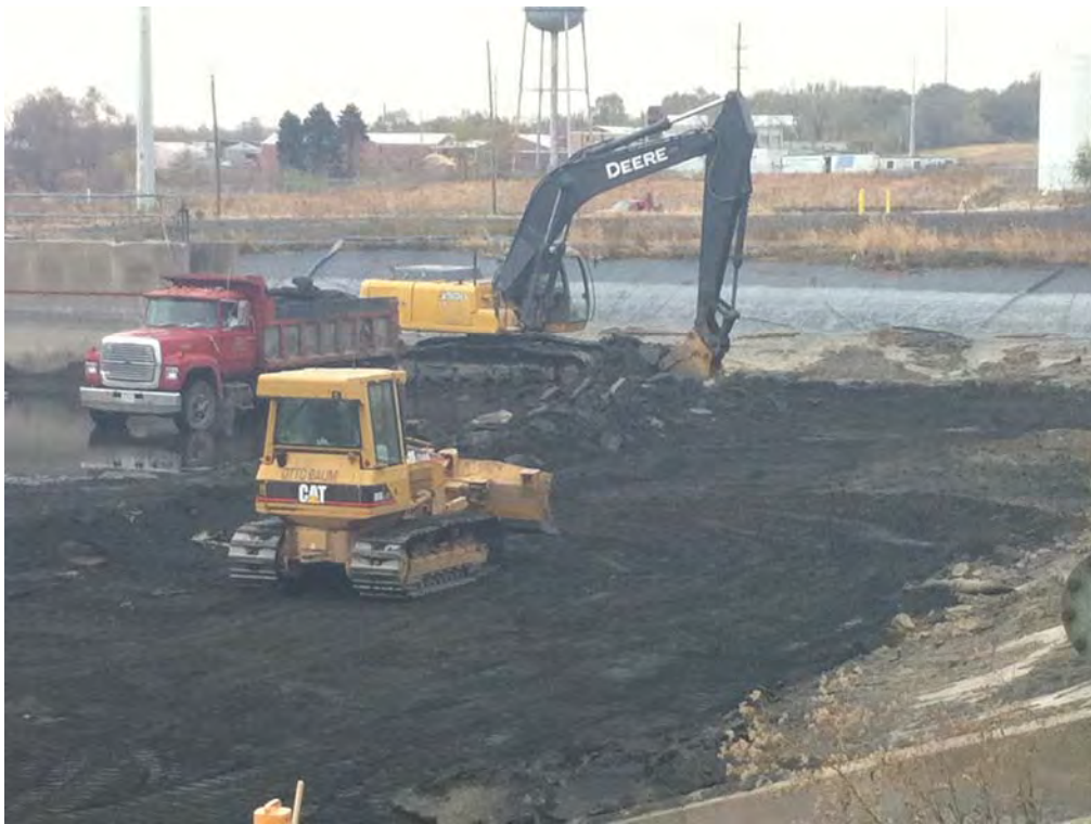
View of pozopac removal and subgrade preparation.
