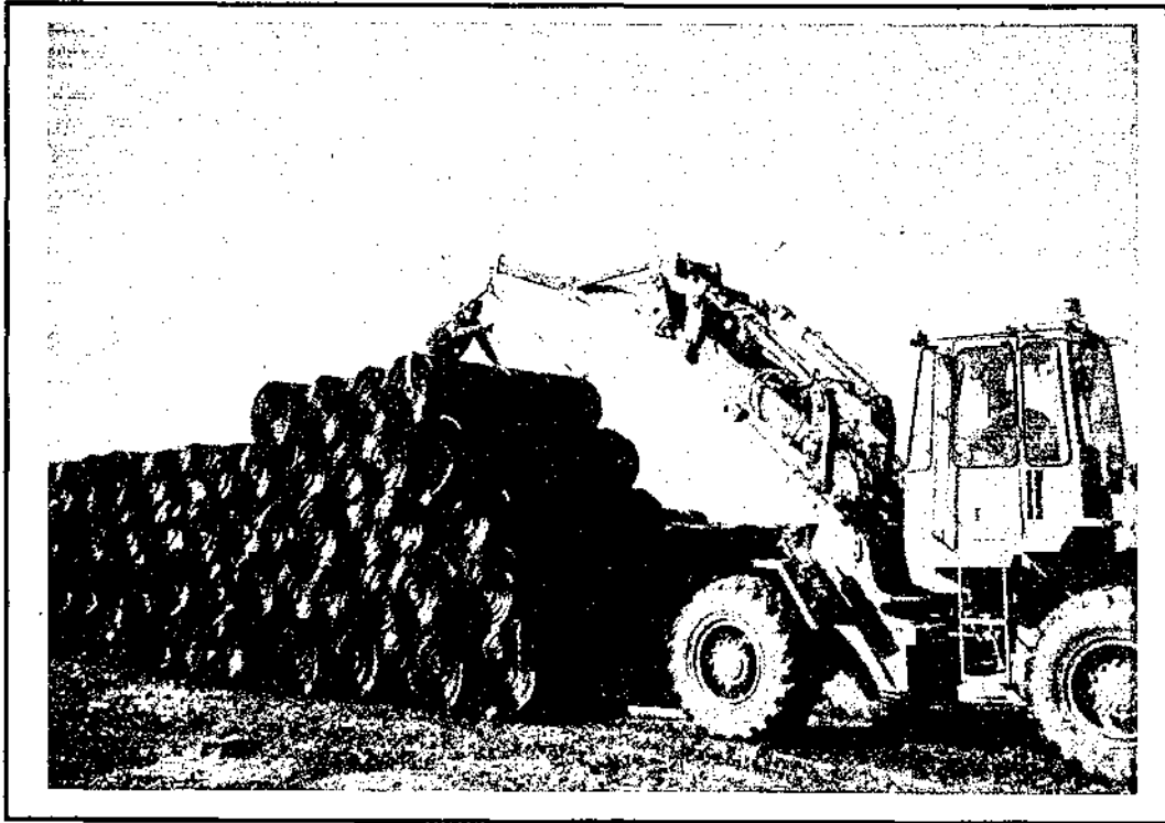
Figure 6.10 - Geonets Being Temporarily Stored at the Job Site
