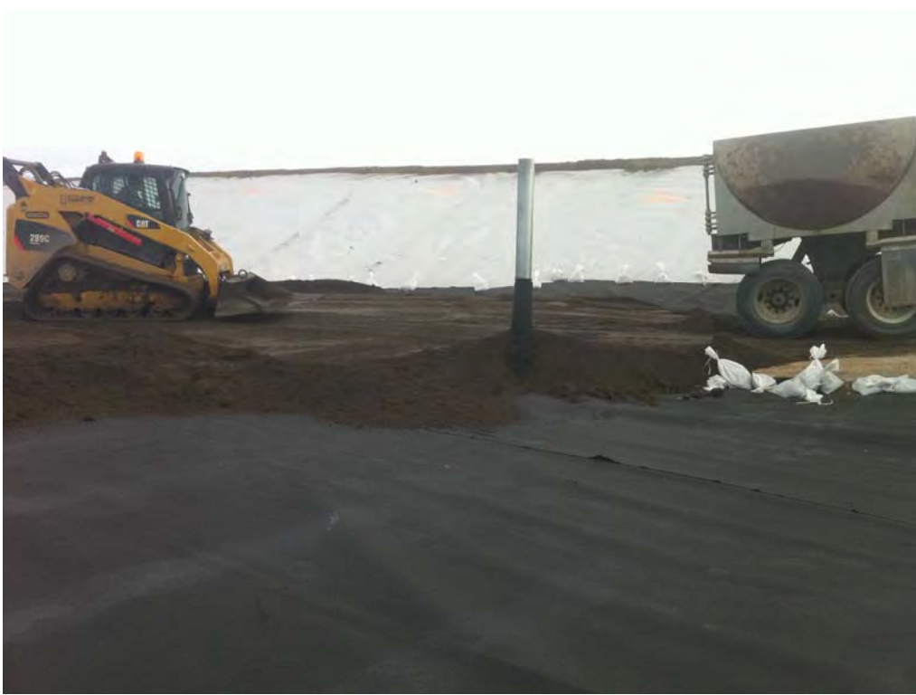
View of liner placement of cushion layer sand.
