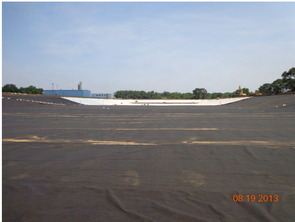
Extent of geosynthetics installation at close of day (looking north)
