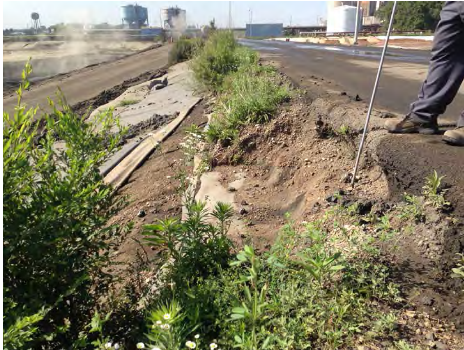
South-facing view of eastern slope, Poz-O-Pac and transition in good condition, some ash remains that will be removed
