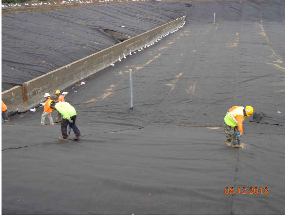
Heat bonding geotextile seams (looking east).
