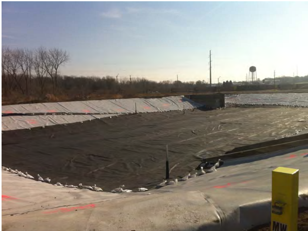
View of finished liner with finished 12 oz geotextile .
