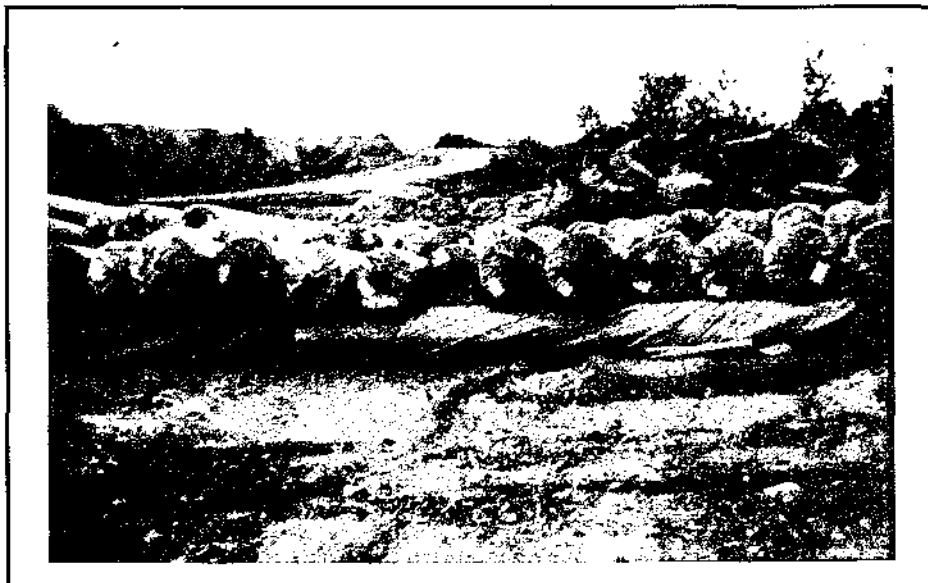
(b) Storage at Field Site
