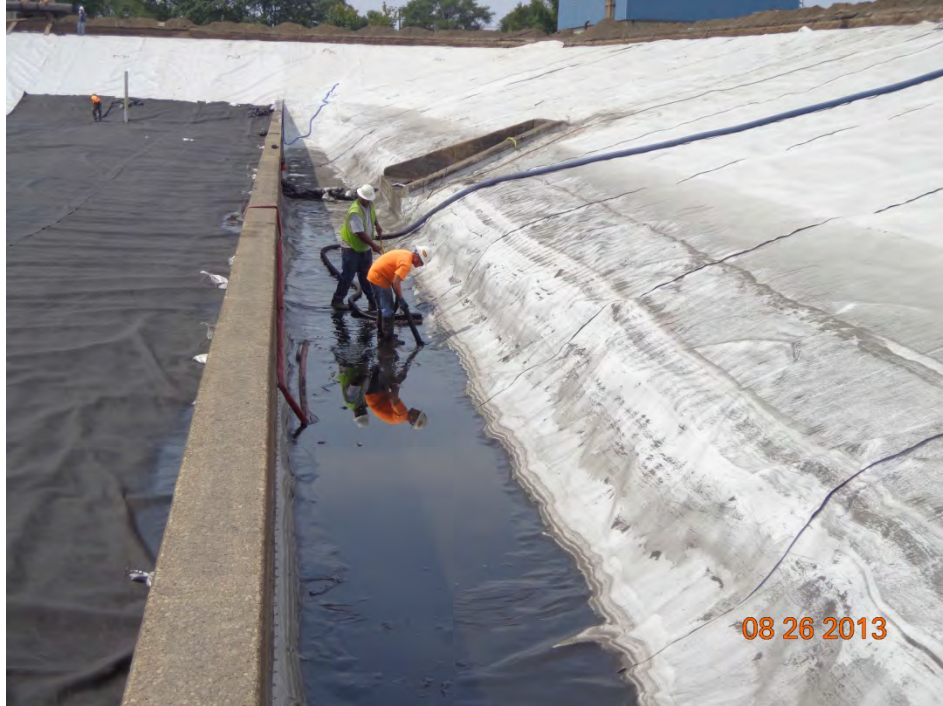
Dewatering the flooded basin (looking west)
