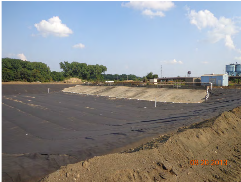
Extent of fabric deployment to the south (looking southeast)
