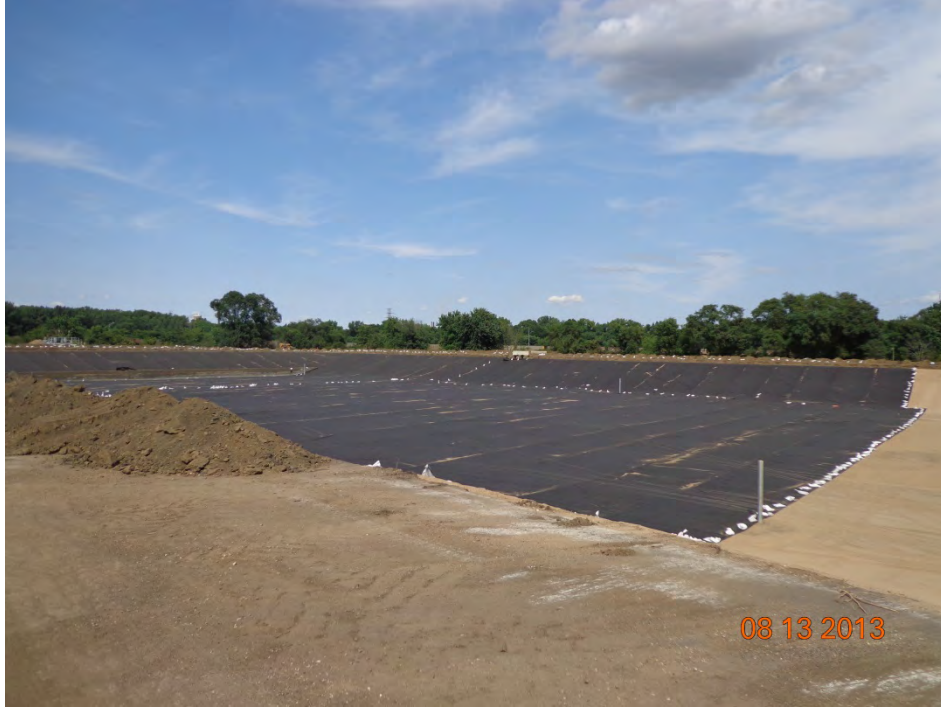
Extent of the day's nonwoven geotextile installation (looking northeast).
