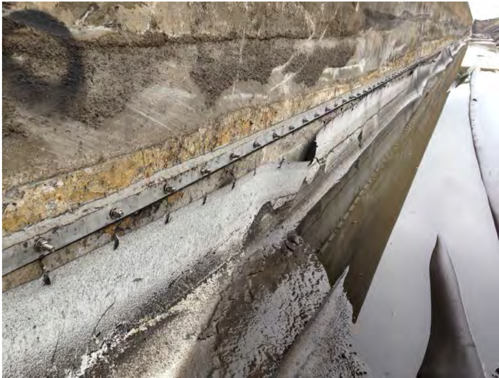
Damaged connection to batten strip on north side of weir wall, facing southwest
