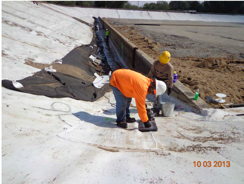
Vacuum testing a new patch along the weir wall (looking east)
