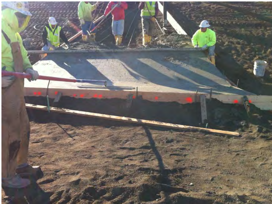
View of the construction of the concrete apron.
