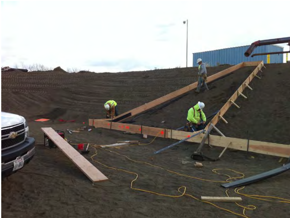
View of the concrete apron forms. Note HDPE weld strip.
