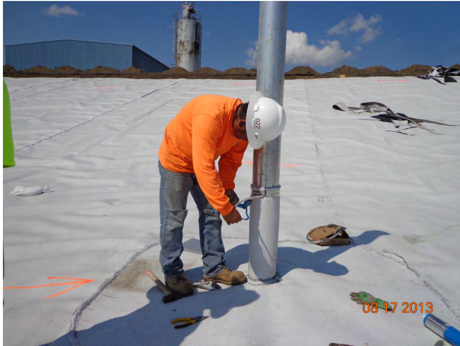
Geomembrane boot installation on a riser (looking west)
