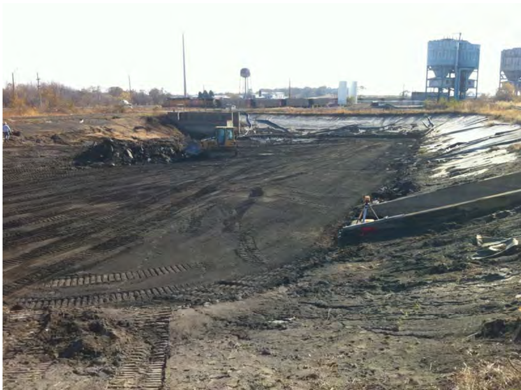
View of pozopac load out and subgrade preparation.
