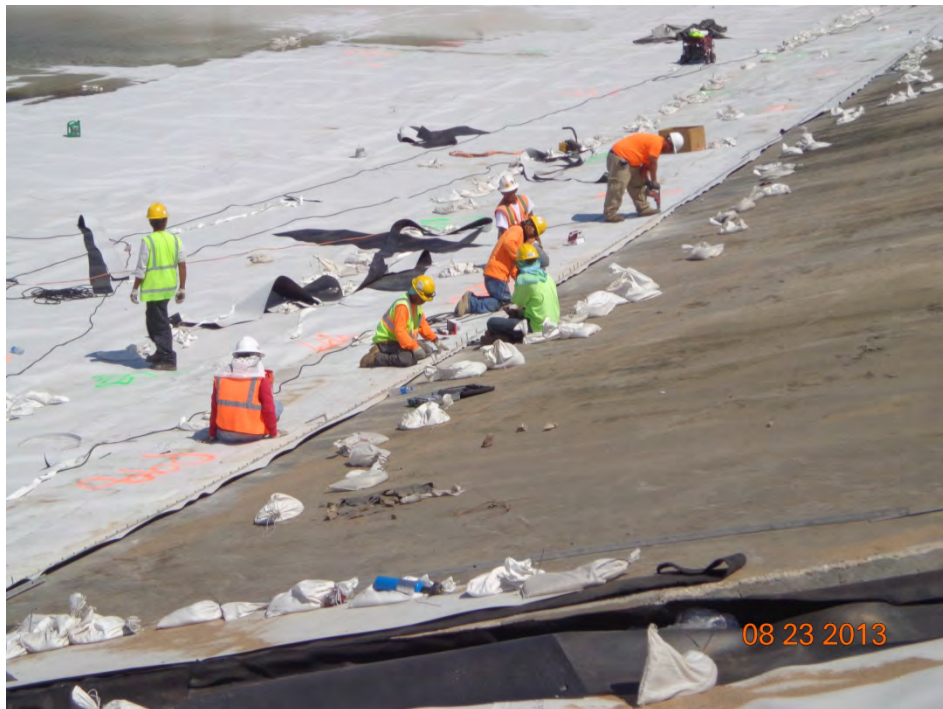
Geomembrane detail work along the inlet ramp (looking northeast)
