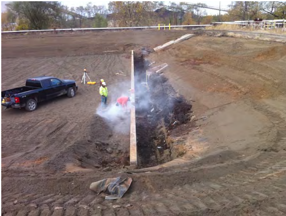
View of excavated weir wall during steel gate removal.
