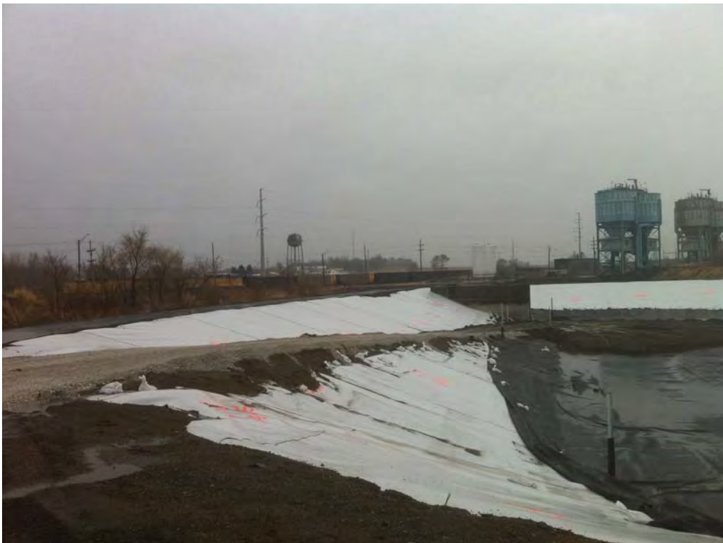
View of finished ramp into bypass basin.
