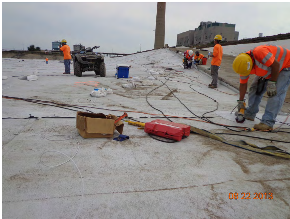
Repairing geomembrane along the ramp (looking southwest)
