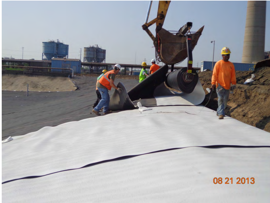
Geomembrane liner deployment towards the south of the basin (looking south)
