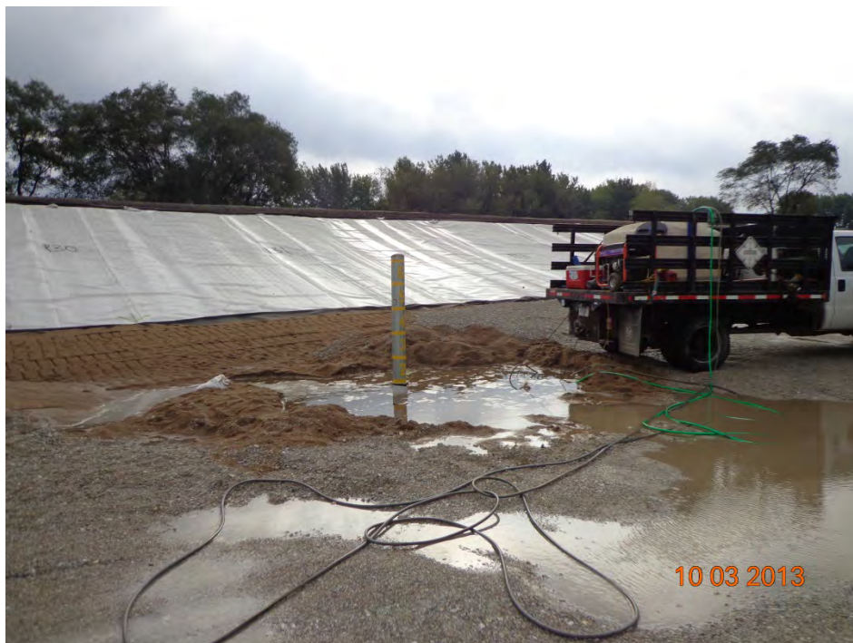
Pumping water from riser pole after the rain (looking southeast)
