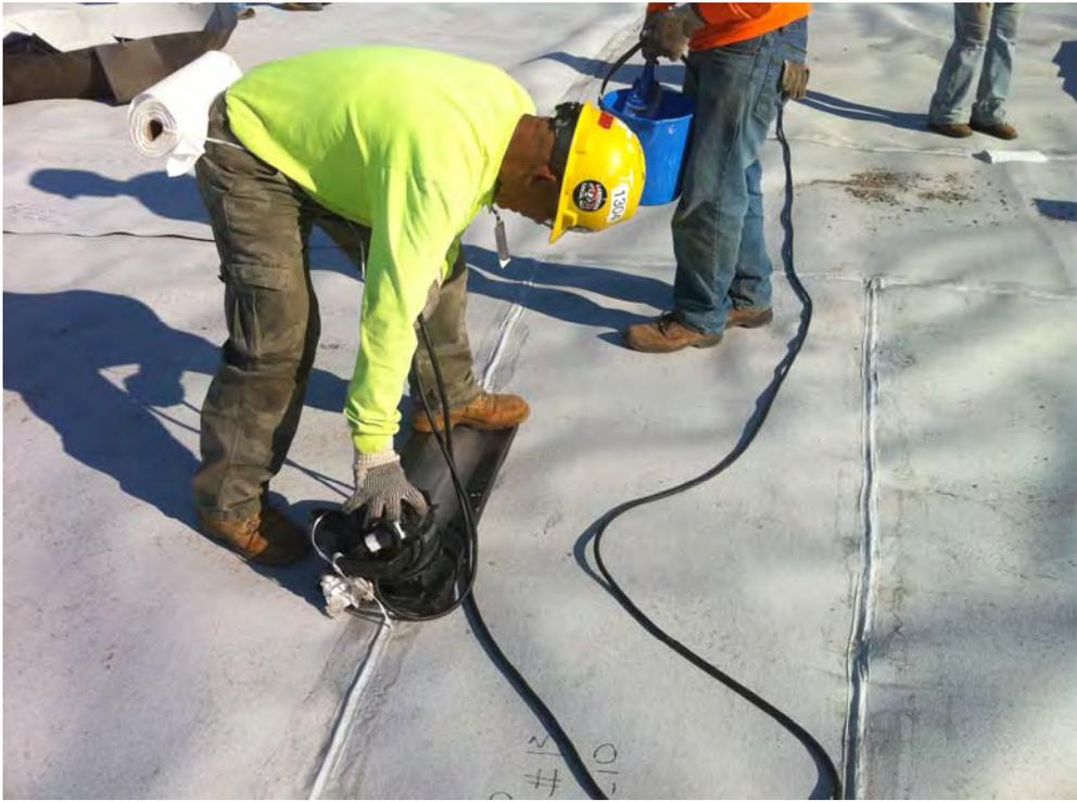
View of extrusion seaming vacuum testing.
