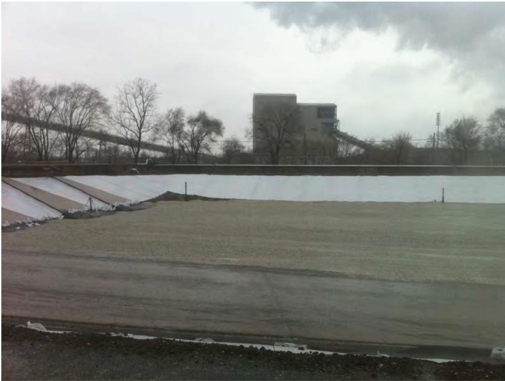
View of warning layer in the southern end of basin where additional cleanup and finishing is required.
