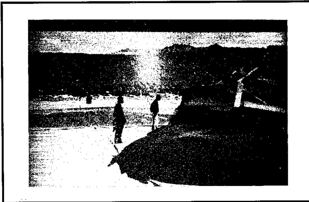
Figure 3.26 - Advancing Primary Leachate Collection Gravel in "Fingers" Over the Deployed Geomembrane
