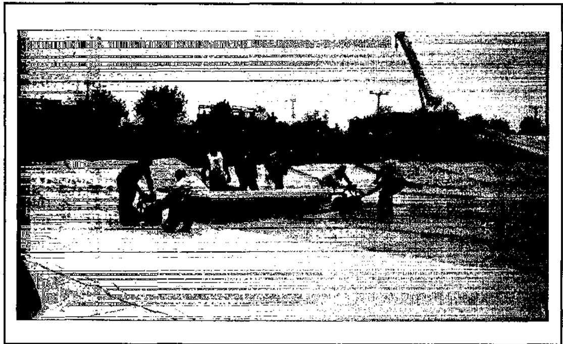
Figure 4.6(b) - Field Deployment of a GCL on an Underlying Geosynthetic
