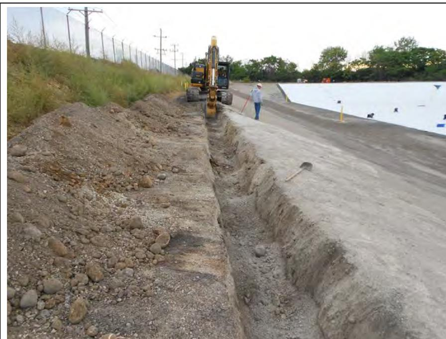
**Installation of geotextile over the remaining pond area, looking northwest**
