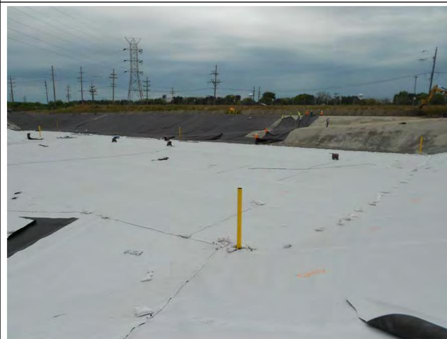
**Non-destructive air testing fusion welded geomembrane seams, looking northwest**
