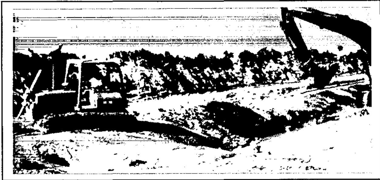
Figure 7.12 - Mixing Backfill with Bentonite Slurry.
