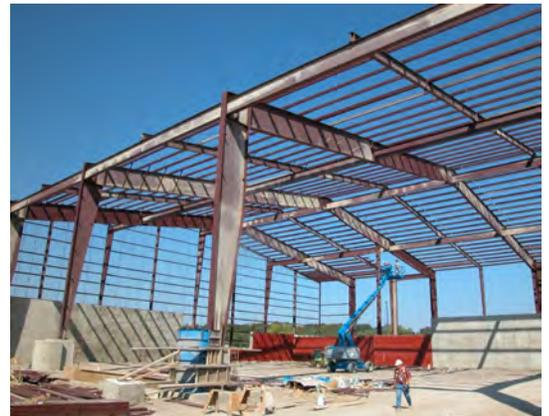
*Concrete push walls and sturdy construction are needed at solid waste transfer stations. High ceilings allow for the opening of compactor trucks and dump beds within the containment of the building. This new construction was at the Tazewell Transfer Station, that opened in January 2008.*
