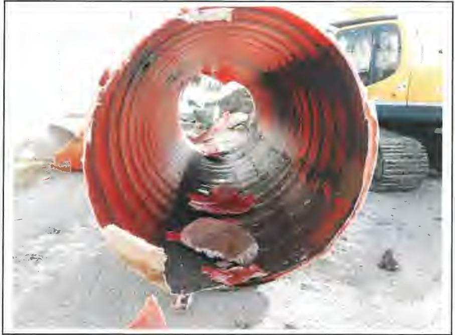
**DESCRIPTION:** UST opened and prepared to be cut/crushed and properly disposed of.
