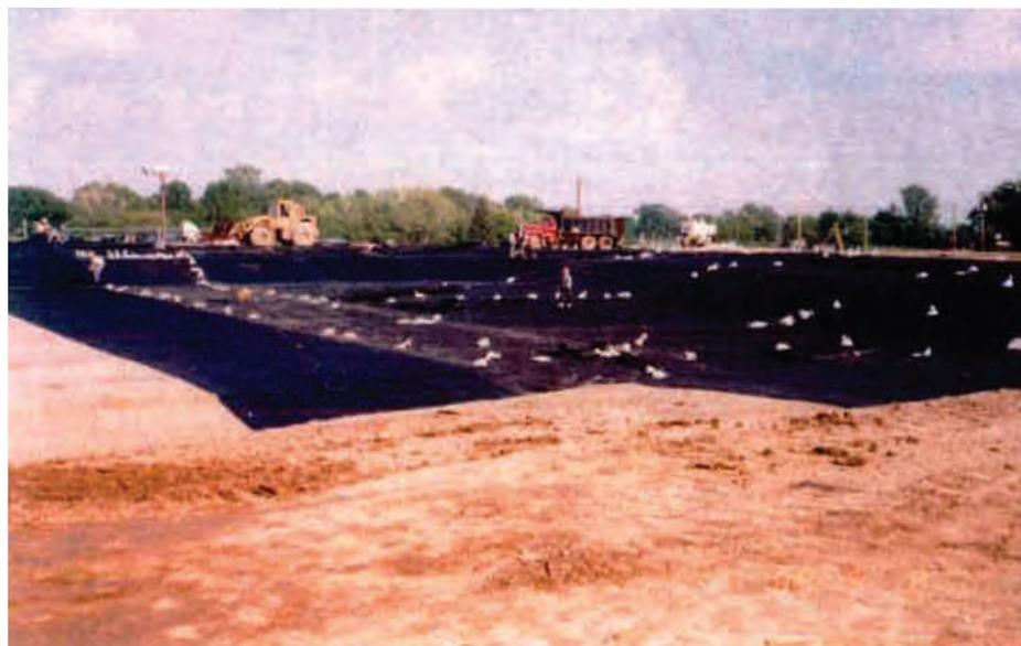
FIGURE 1.2 Geomembrane cover placed over contaminated ground as part of a RCRA Corrective Action at Love Canal in New York state in 1989. SOURCE: Scott Parkhill, Miller Springs Remediation Management, Inc.
