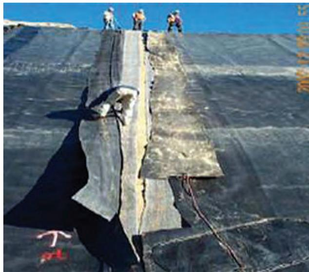
FIGURE 4.2 GCL seam separation at a California landfill. SOURCE: County of Riverside (2004).
