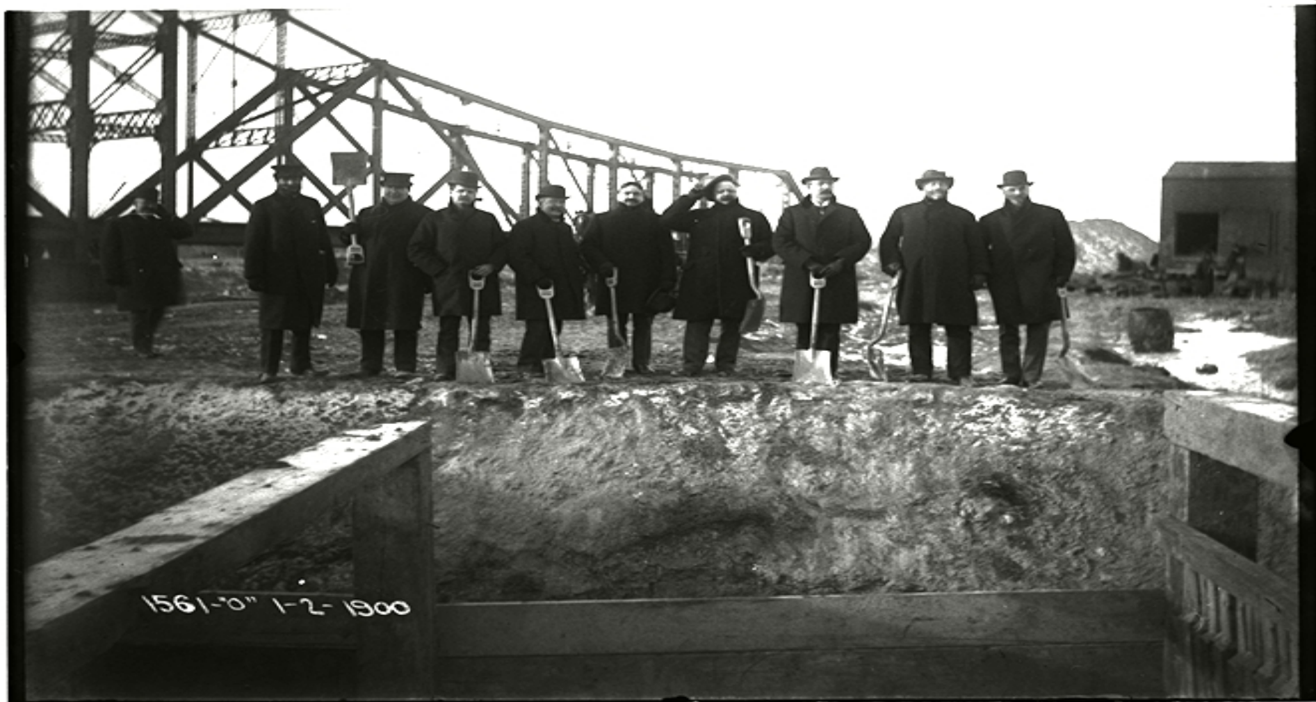
1.2.1900 - SDC trustees preparing to symbolically dig a channel to connect the Collateral Channel to the excavated CSSC to start the filling process.
